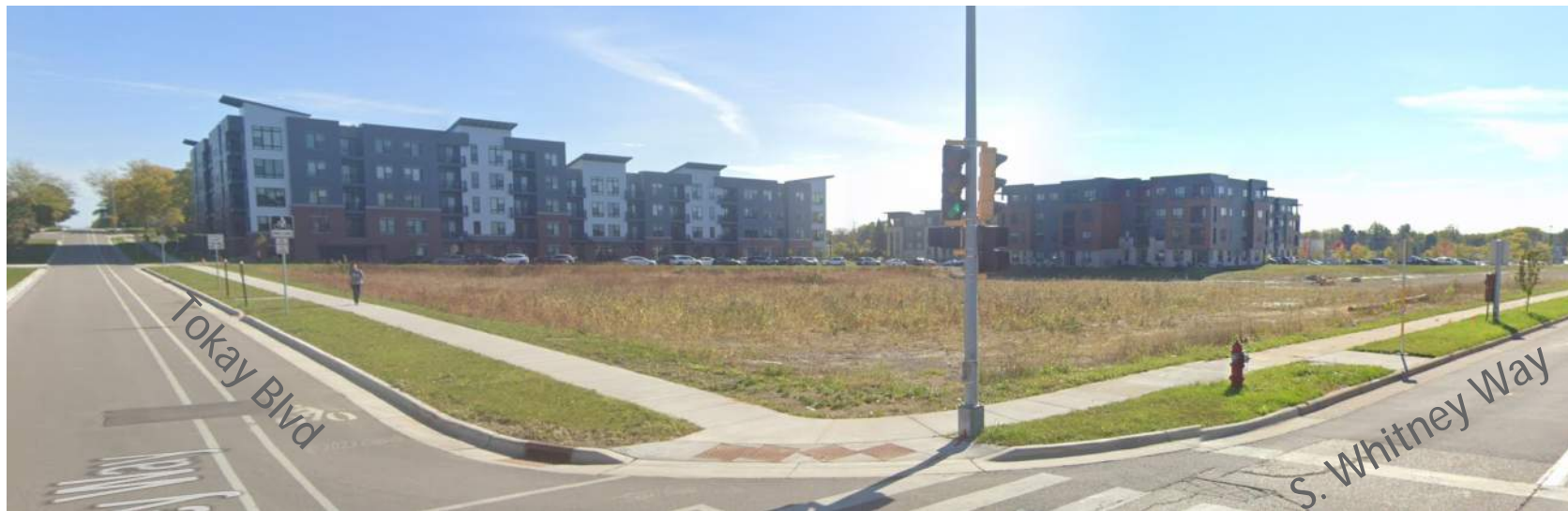
C - View looking southeast
