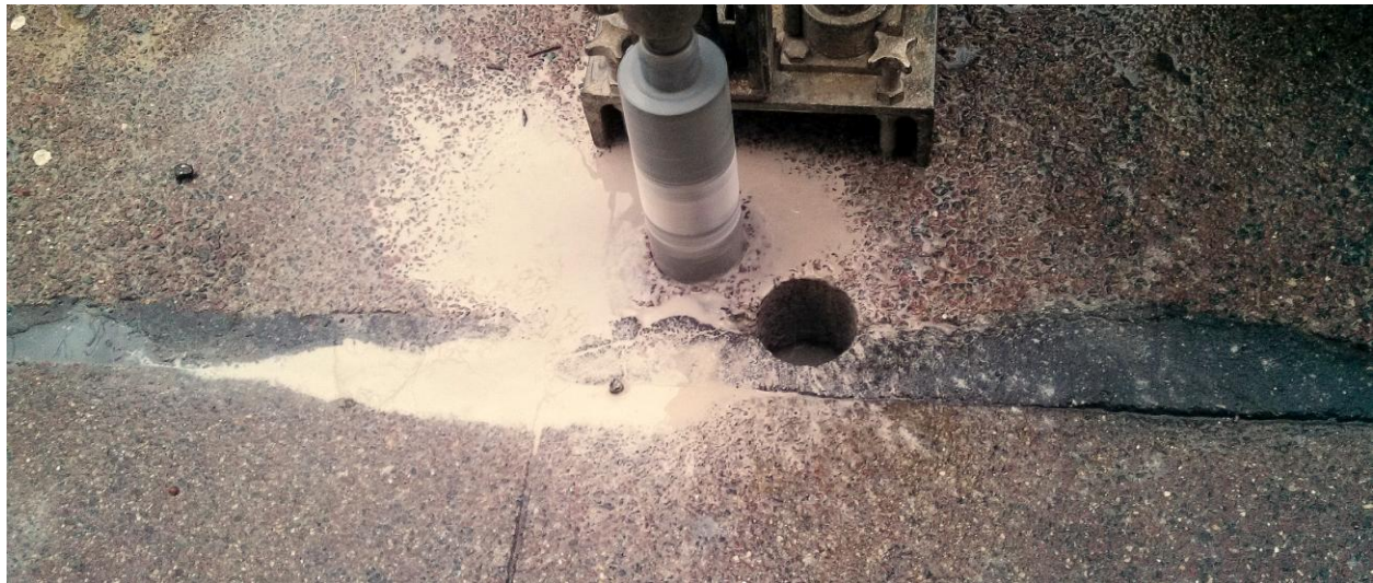
Figure 4. The location of cores showing the deterioration and which were subjected to laboratory testing.
