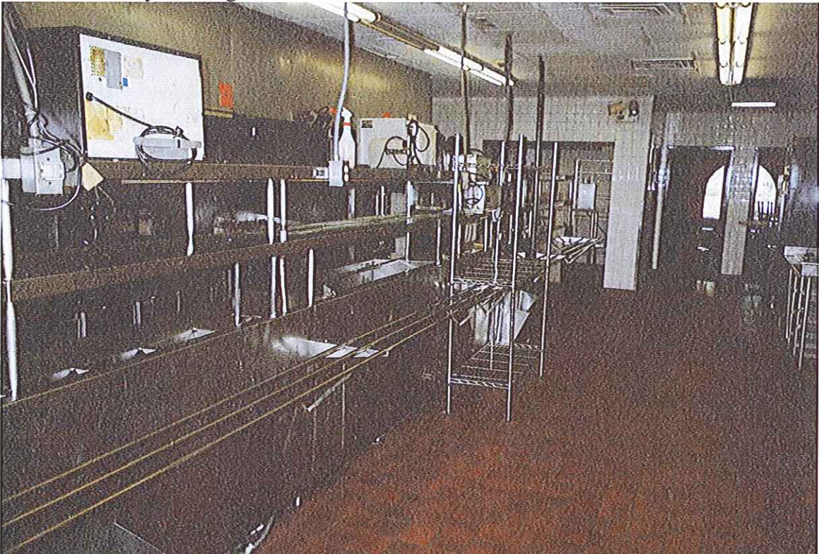
Figure 18 - Main kitchen area of the Chi Chi's Restaurant building.
