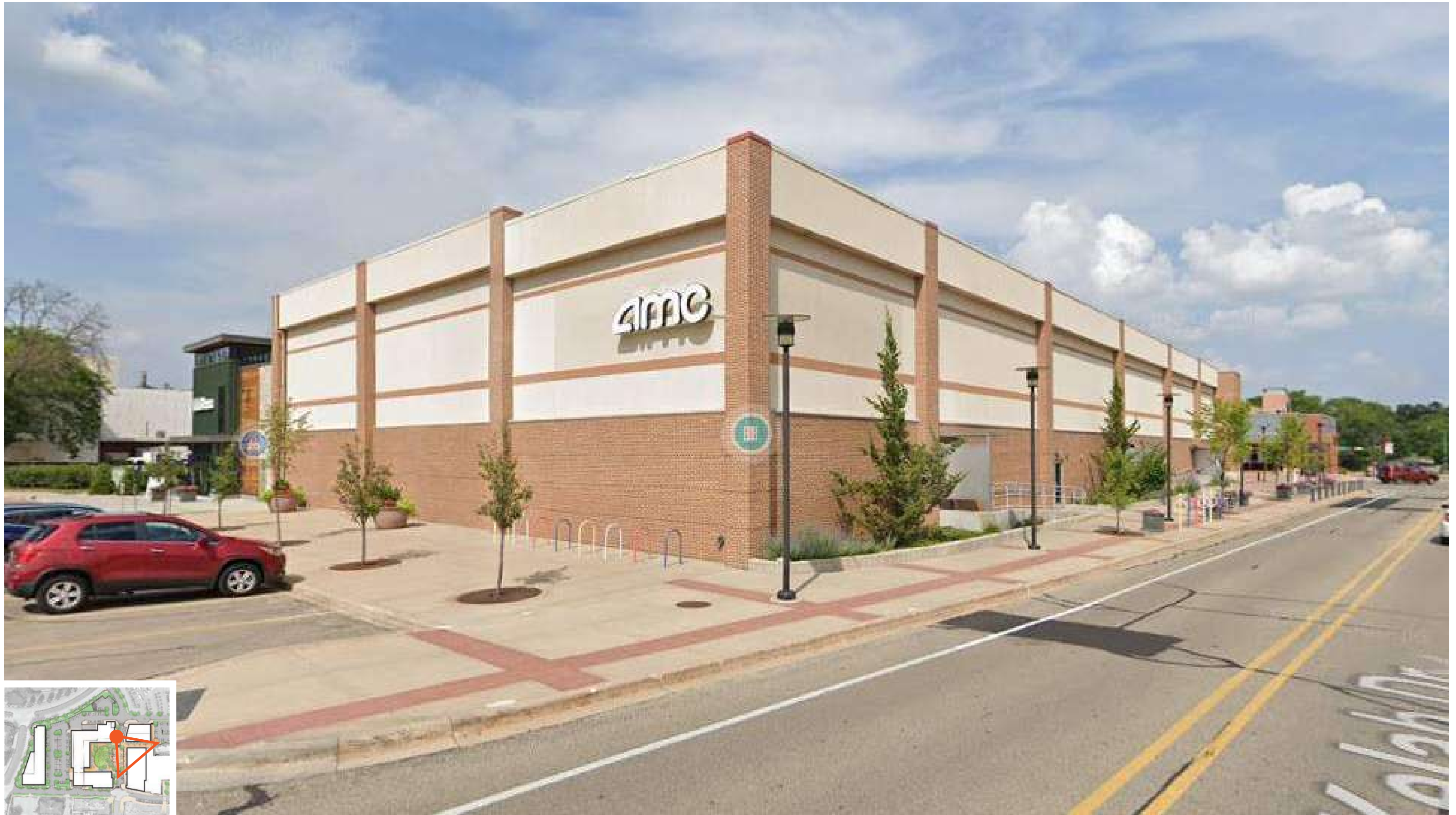
BUILDING 100 - SOUTHWEST PHOTO OF EXISTING
