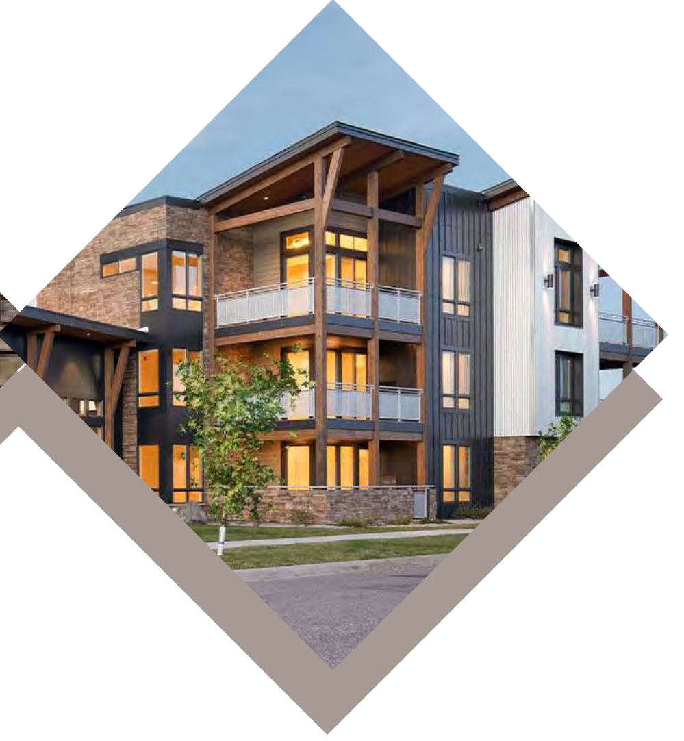
WOOD BEAMS & COLUMNS
