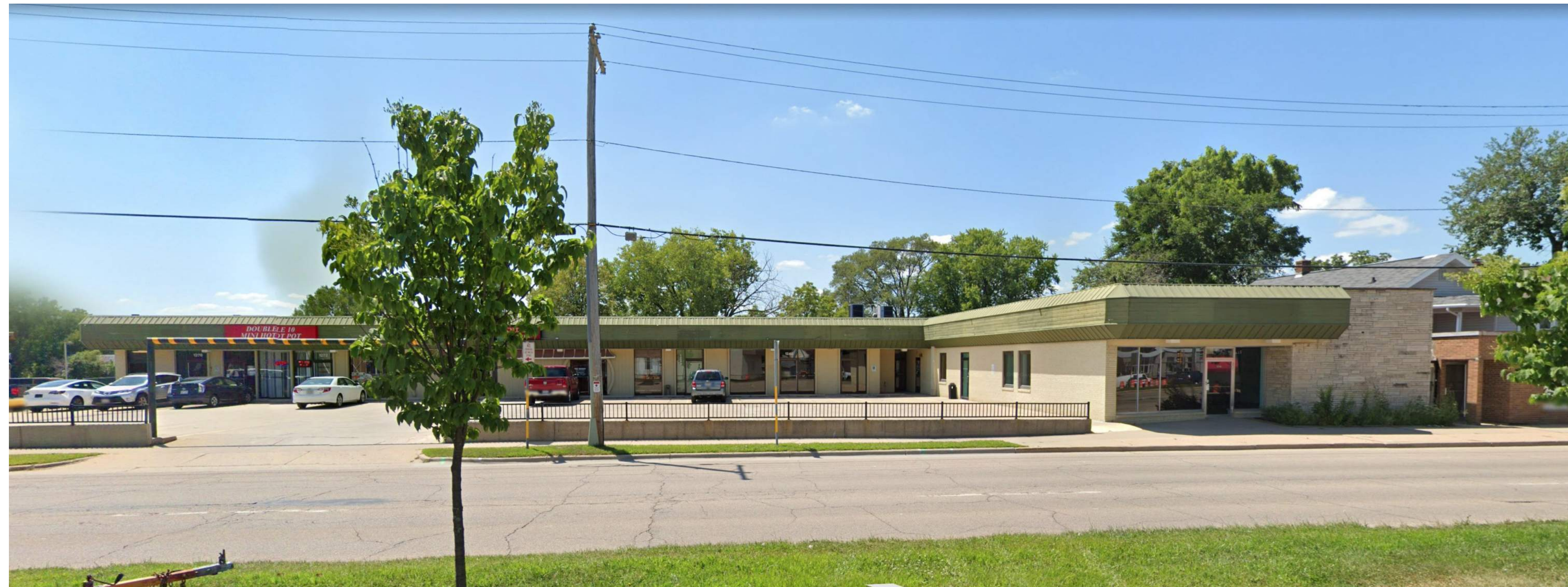
Project Site | 1224 S. Park St. | Wingra Creek Center
