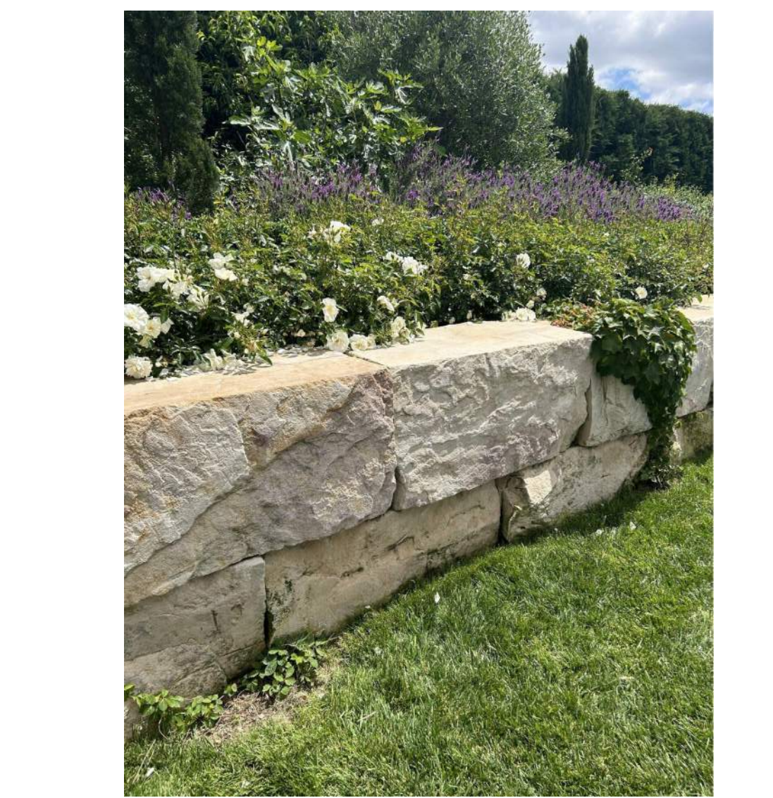
3 DETAIL- LIMESTONE BLOCK WALL (WL-02) NTS P-26.109-02
