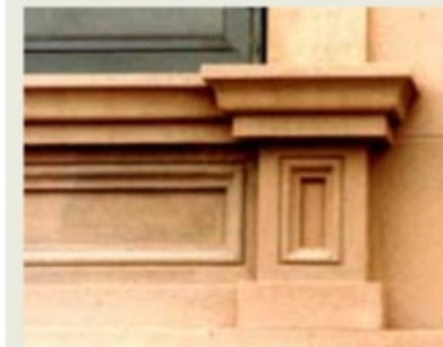
Same detail, after stucco repair. Simplified, but met the Standards.
