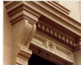
Detail, doorway brackets.
