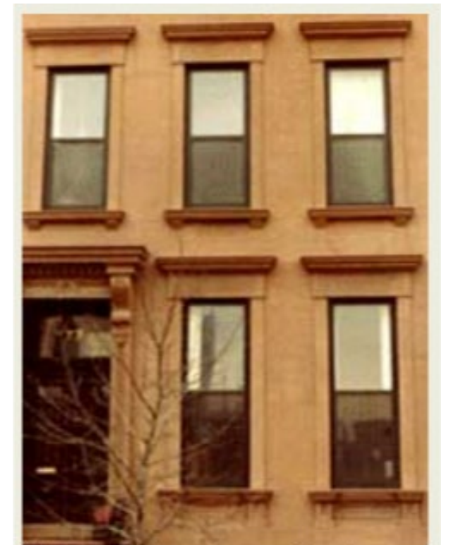
"Brownstone" rowhouse after stucco repair.
