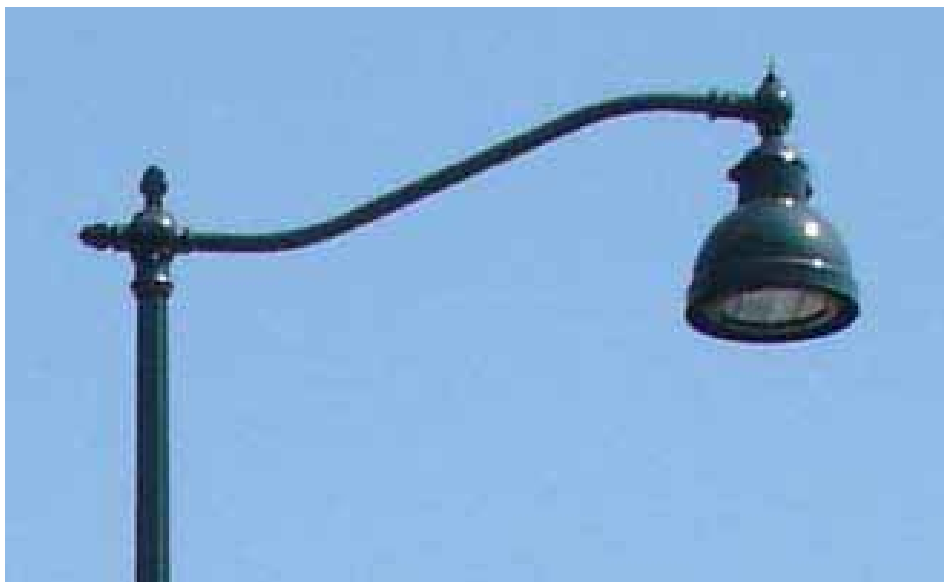
Cut off lighting on E Washington Avenue. Image: City of Madison Traffic Engineering
