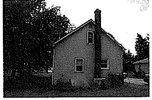
IMG_0967 4706 North Side
