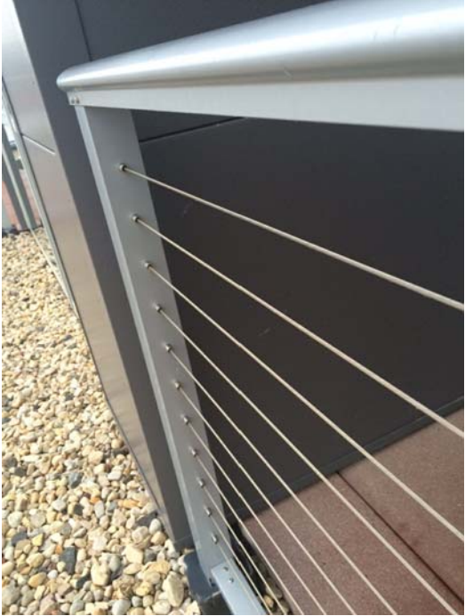
ALUMINUM AND STAINLESS STEEL RAILING
