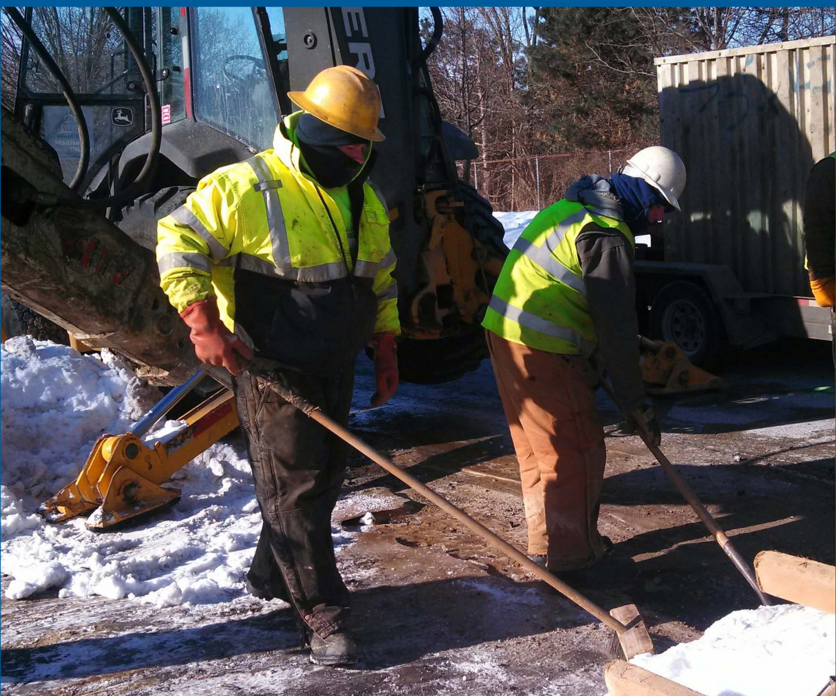
MWU CREW WORKING IN SUBZERO TEMPERATURES DURING THE POLAR VORTEX. JANUARY 6, 2014
