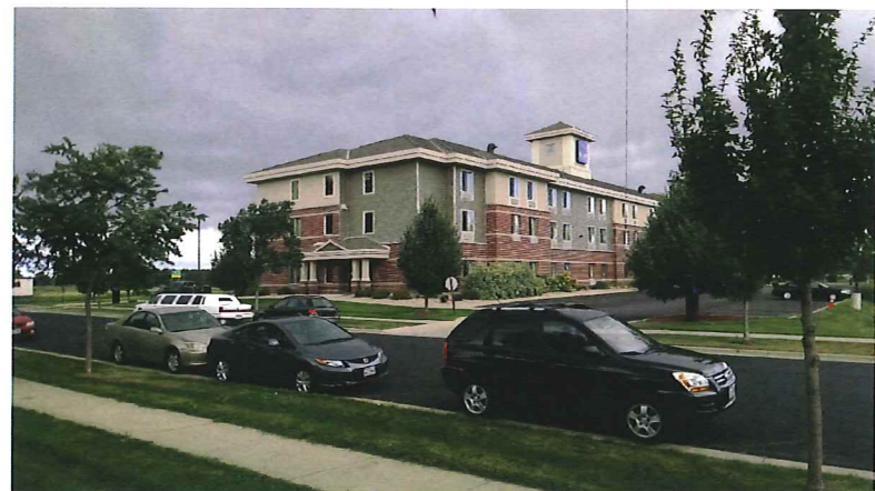
Existing Building From South-East
