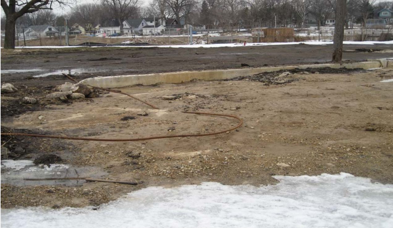
Abandoned Foundation March 17, 2008
