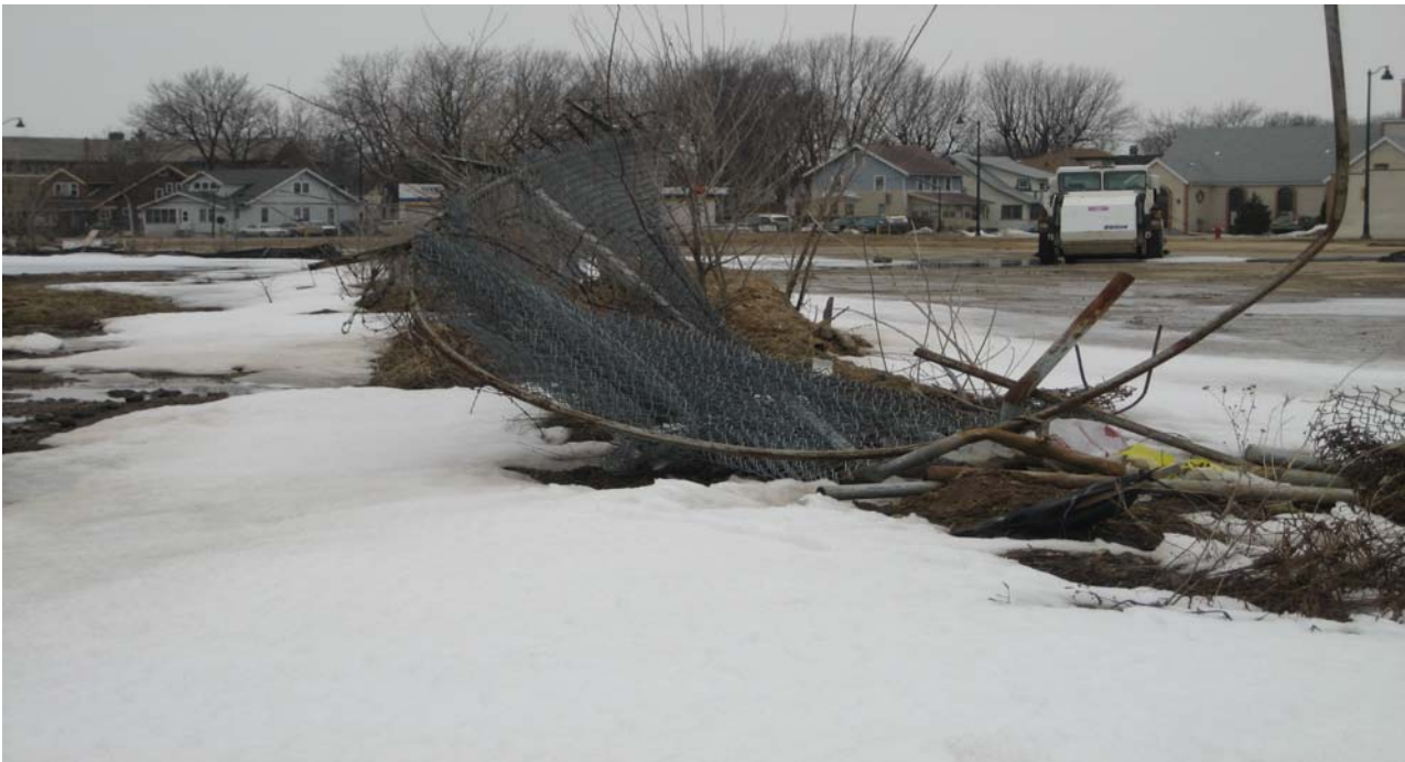
More Leaning Fence March 17, 2008
