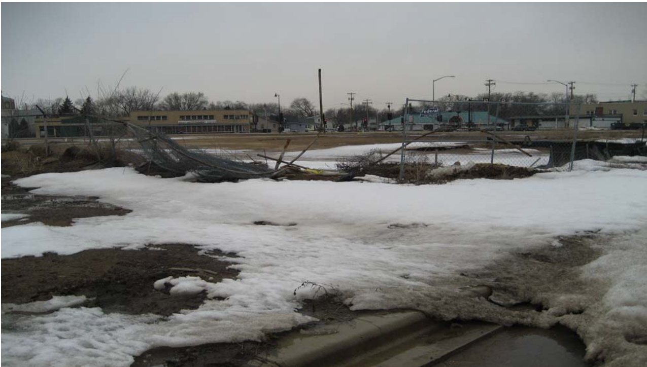
Broken Fence March 17, 2008
