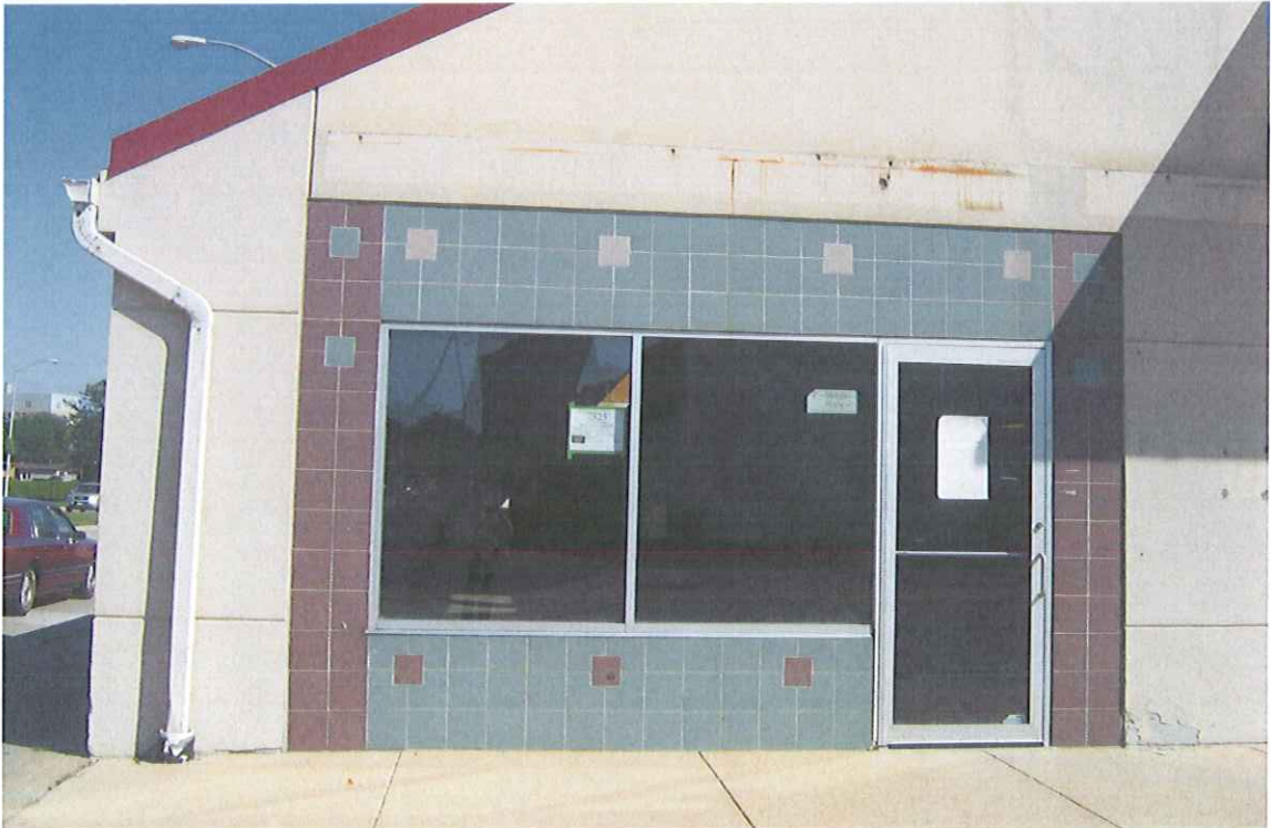
WEST SIDE OF SUBJECT SITE, POSSIBLE ENTRANCE LOCATION
