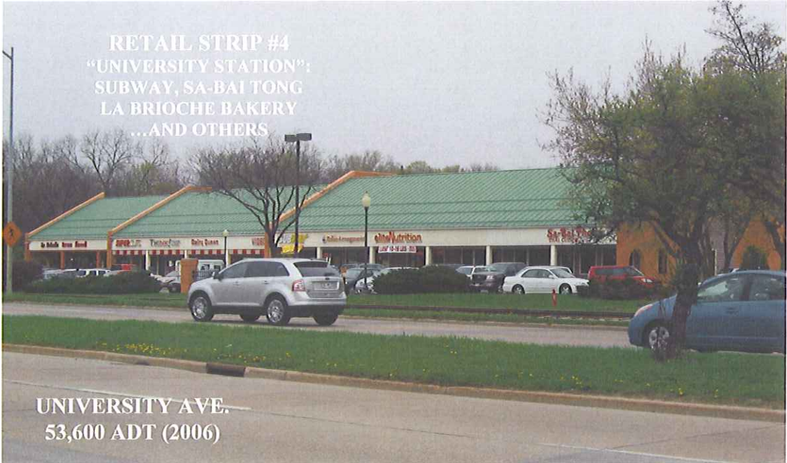
1/10 MILE WEST ON UNIVERSITY AVE, LOOKING NORTH
