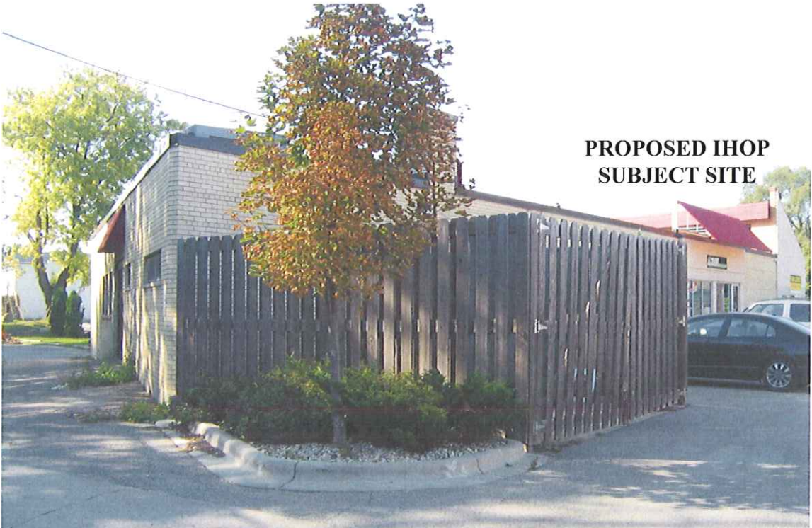
SOUTH SIDE (BACK) OF SUBJECT PROPERTY AT FRANKLIN COURT
