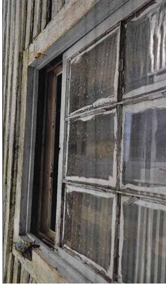
[231] (a) This deteriorated historic wood window was repaired and retained (b) in this rehabilitation project.
