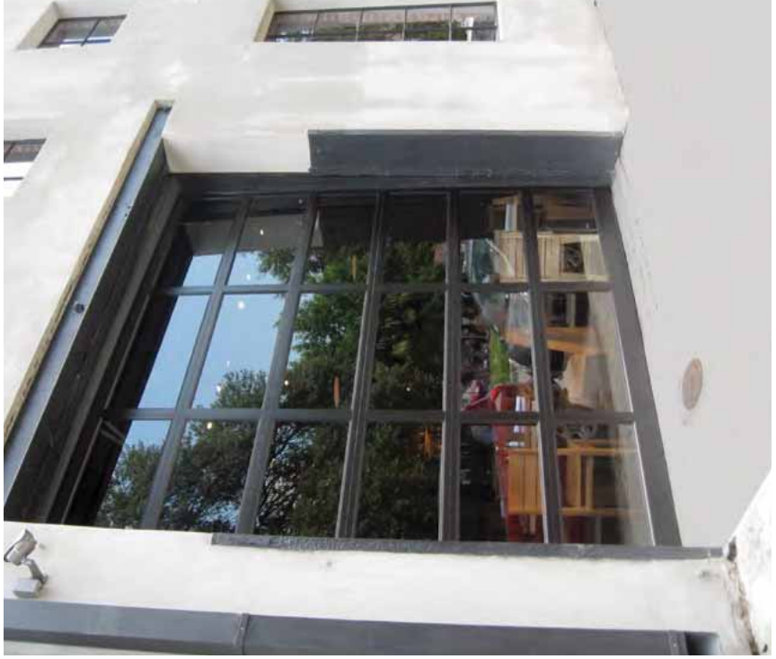
[25] The new infill designs for the garage door openings in this commercial building (a) converted for restaurant use and in this mill building (b) rehabilitated for residential use are compatible with the historic character of the buildings.
