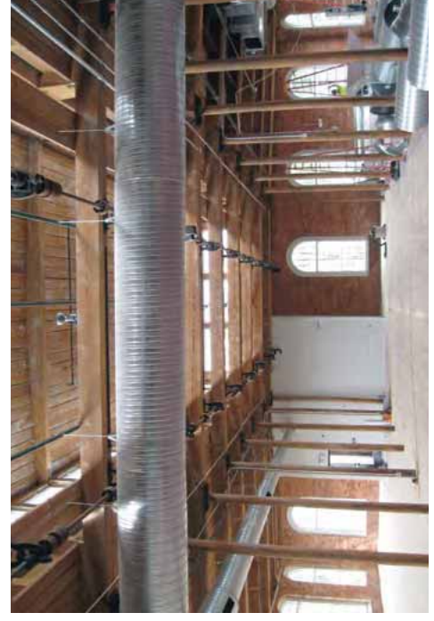
[39] Leaving the ceiling structure exposed and installing exposed ductwork where it does not impact the windows, are appropriate treatments when rehabilitating an industrial building for another use.
