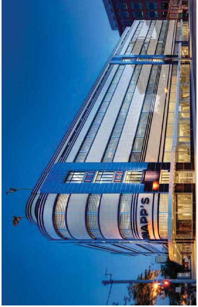
[7] (a) J.W. Knapp's Department Store, built 1937-38, in Lansing, MI, was constructed with a proprietary material named "Maul Macotta", made of enameled steel and cast-in-place concrete panels. Prior to its rehabilitation, a building inspection revealed that, due to a flaw in the original design and construction, the material was deteriorated beyond repair. The architects for the rehabilitation project devised a replacement system (b) consisting of enameled aluminum panels that matched the original colors (c). Photos and drawing (a-b): Quinn Evans Architects; Photo (c): James Haefer Photography.
