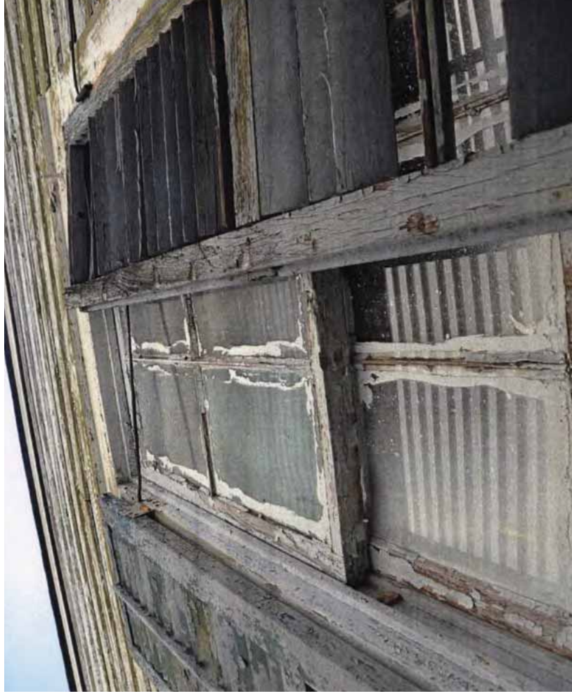
[11] Old and brittle glazing putty should be removed carefully before reputtying to keep window glazing weathertight.
