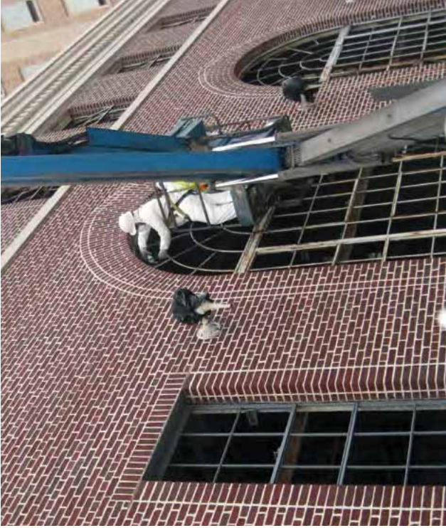
[57] Workers wear protective clothing while removing lead paint from metal features.
