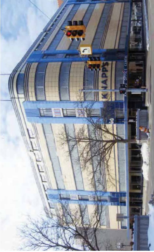
[7] (a) J.W. Knapp's Department Store, built 1937-38, in Lansing, MI, was constructed with a proprietary material named "Maul Macotta", made of enameled steel and cast-in-place concrete panels. Prior to its rehabilitation, a building inspection revealed that, due to a flaw in the original design and construction, the material was deteriorated beyond repair. The architects for the rehabilitation project devised a replacement system (b) consisting of enameled aluminum panels that matched the original colors (c). Photos and drawing (a-b): Quinn Evans Architects; Photo (c): James Haefer Photography.
