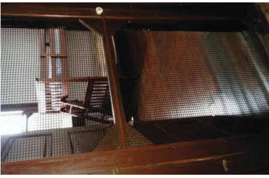
[31] An interior screen door at the entrance to individual apartments is a historic feature traditionally used to help circulate air throughout the building.
