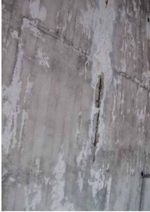
[5] Rebars in the reinforced concrete ceiling have rusted, causing the concrete to spall. The rebars must be cleaned of rust before the concrete can be patched.
