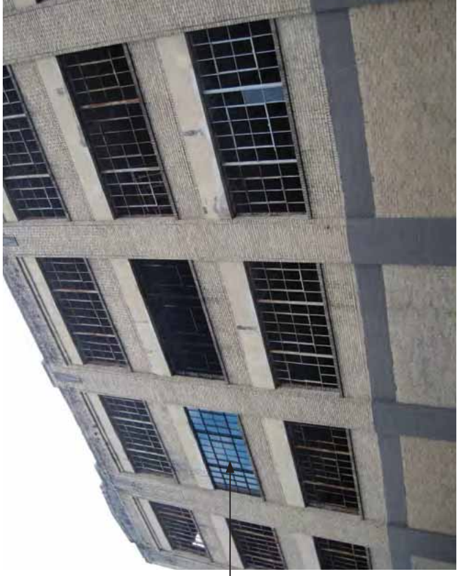
[19] Installing a mockup of a proposed replacement window can be helpful to evaluate how well the new windows will match the historic windows that are missing or too deteriorated to repair.
