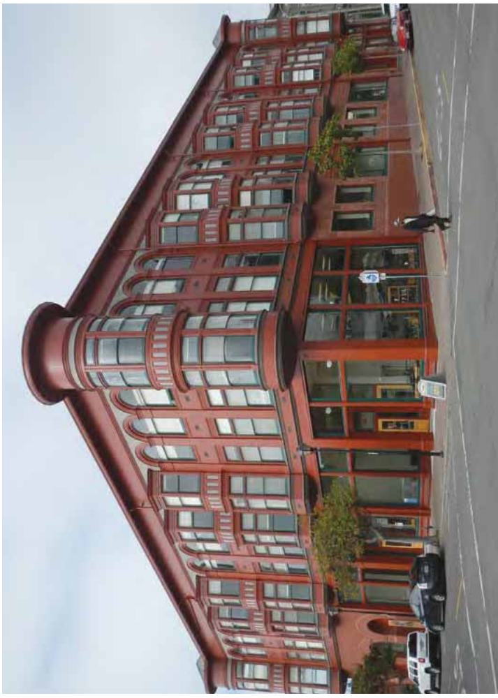
[32] (a-b) The rehabilitation of the 1892 Carson Block Building in Eureka, CA, for its owner, the Northern California Indian Development Council, included recreating the missing corner turret and sensitively introducing seismic reinforcement (C) shown here (opposite page) in a secondary upper floor office space. Photos: Page & Turnbull.
