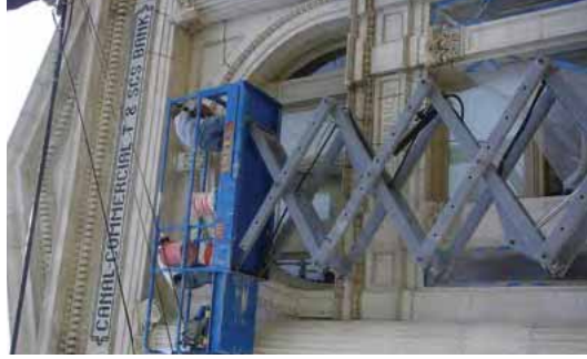
[1] An alkaline-based product is appropriate to use to clean historic marble because it will not damage the marble, which is acid sensitive.
