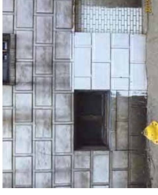
[1] A test patch should always be done before using a chemical cleaner to ensure that it will not damage historic masonry, as in this instance, terra cotta.
