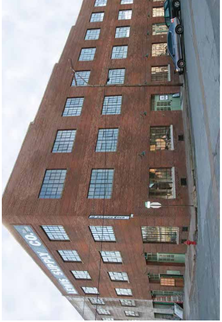
[20 a-d] The original steel windows in this industrial building were successfully repaired as part of the rehabilitation project (left).
