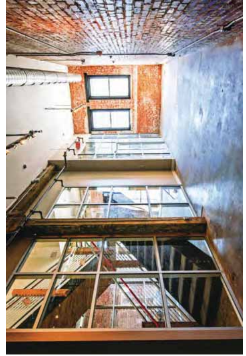
[38] The rehabilitation project retained the industrial character of this historic factory building, which included installation of a fire-rated, clear glass enclosure that allows the stairway, an important interior feature, to remain visible.
