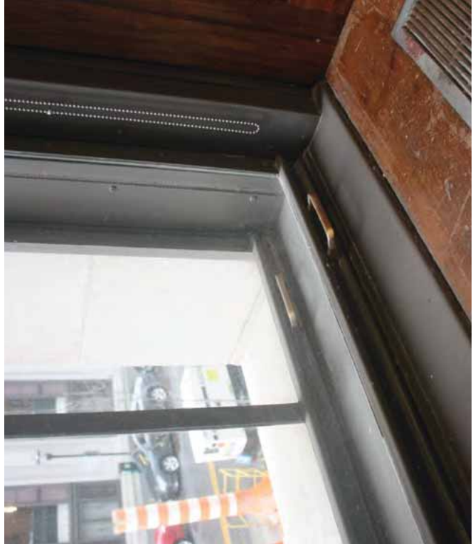
[18] The historic metal storm windows in this 1920s office building were retained and repaired during the rehabilitation project.
