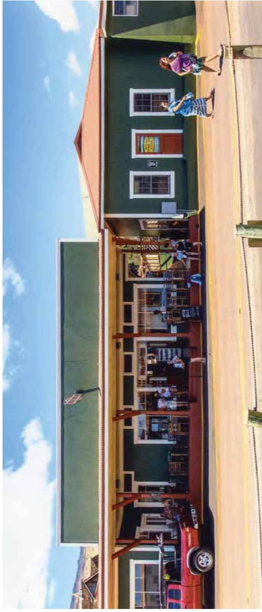
[29] The rehabilitation of the 1910 Māālaea General Store (a), which served the workers' camp at the Wailuku Sugar Company on the Hawaiian island of Maui, included the reconstruction of the original parapet (b).
