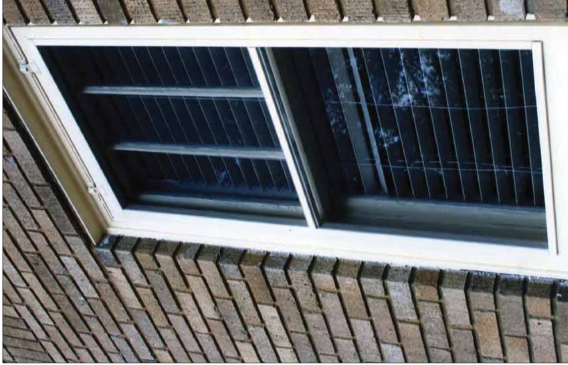
[10] Historic exterior storm windows preserve and help to insulate wood windows.
