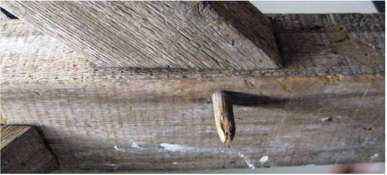
[17] Distinctive examples of traditional construction techniques should be preserved, such as this wooden peg, which is part of the structural system of this late-19th-century warehouse.
