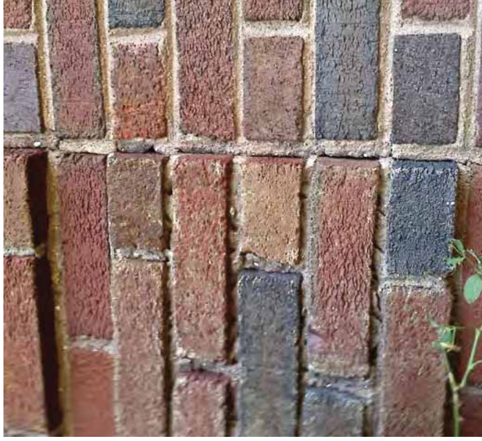
[3] Not Recommended: The white film on the upper corner of this historic brick row house is the result of using a scrub or slurry coating, rather than traditional repointing by hand, which is the recommended method.
