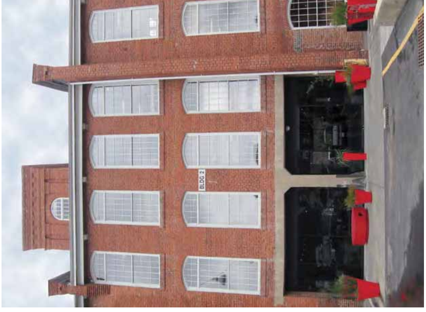
[25] The new infill designs for the garage door openings in this commercial building (a) converted for restaurant use and in this mill building (b) rehabilitated for residential use are compatible with the historic character of the buildings.
