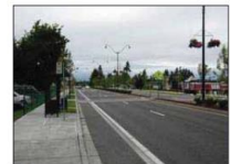
FIGURE 4.18 Separate facilities for transit users, pedestrians, and bicyclists make this an active arterial for many users.
