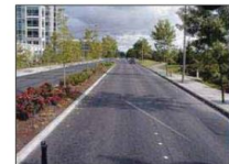
FIGURE 4.16 An example of a four lane road separated by a landscaped median
