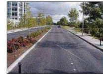
FIGURE 4.16 An example of a four lane road separated by a landscaped median
