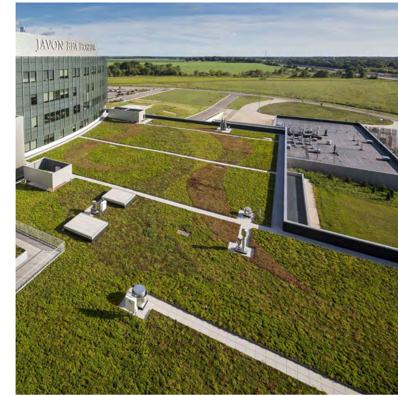
Typical rooftop / penthouse green roof with 2' clear zone around outside edges and mechanical units. Includes additional paver walkways for maintenance access.
