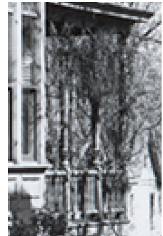
ORIGINAL PORCH RAILING
