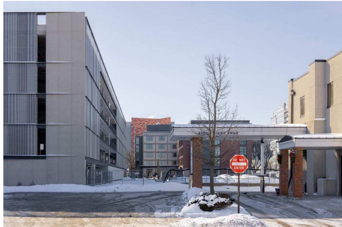
Project site between Madison Credit Union, Phase 1 Parking Ramp, and Hotel Indigo
