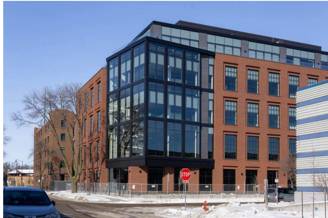
WHEDA Building at E. Main St. and S. Paterson St.
