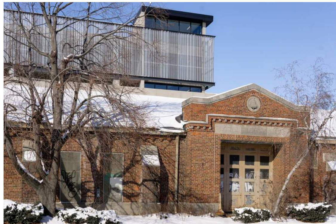
Wisconsin Telephone Company Building at E. Main St. and S. Brearly St.
