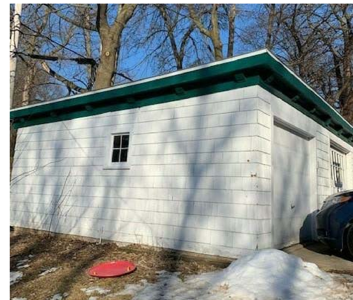
GARAGE SW CORNER
