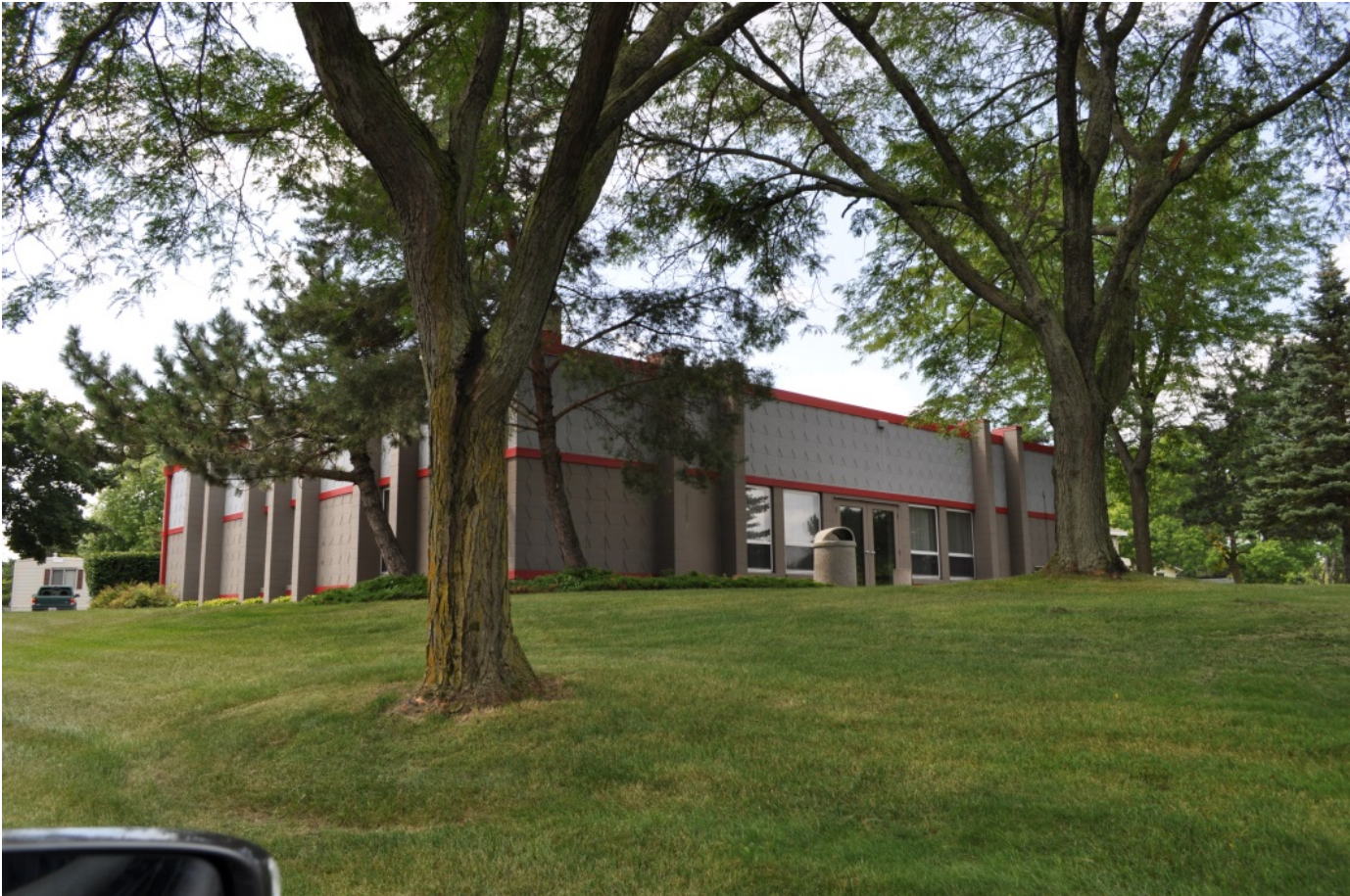
Existing Community Building within Highland Manor Mobile Home Park
