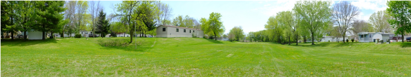
Panoramic of site location – looking west into the site
