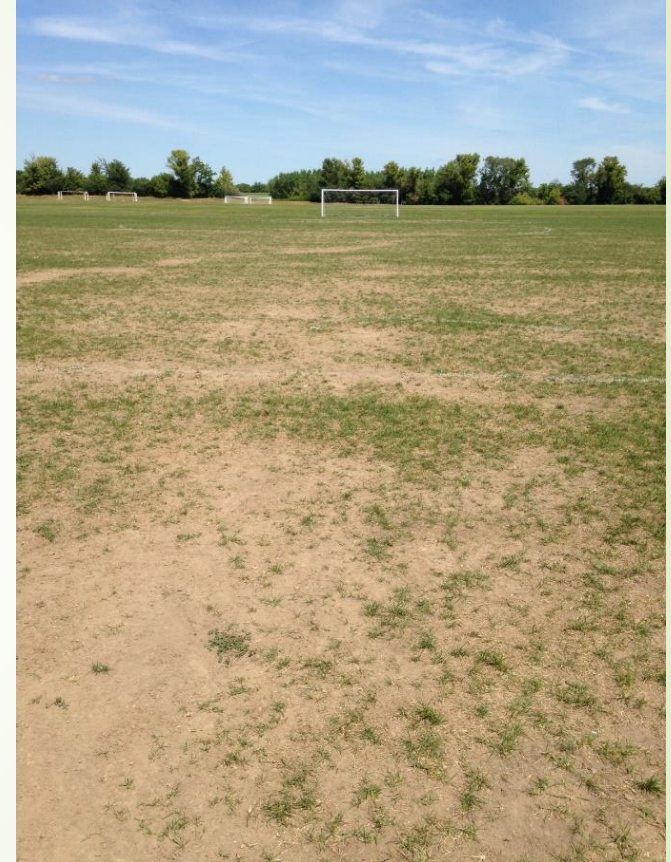
Reindahl Park -- 2014 damage as a result of over-use and compacted soils. Very thin turf that is not safe for play.
