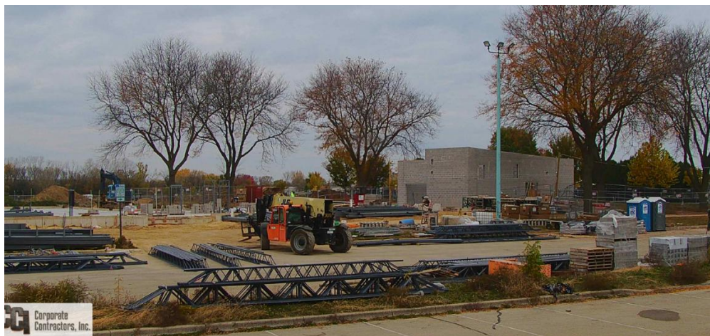
3 Steel on site at the Imagination Center. Photo credit: CCI.
