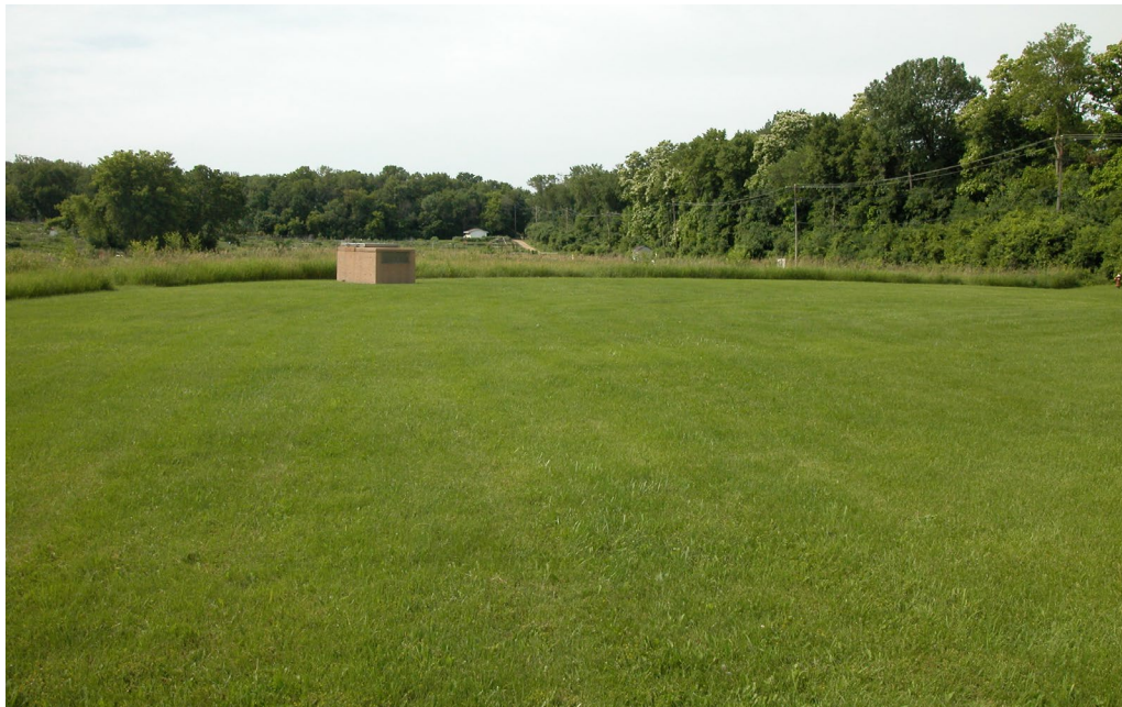
The buried reservoir: facing south
