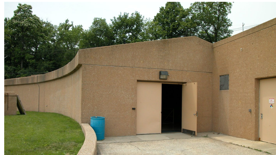
The well house entrance: facing west
