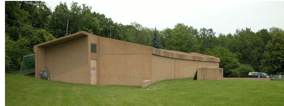
The well house: facing north
