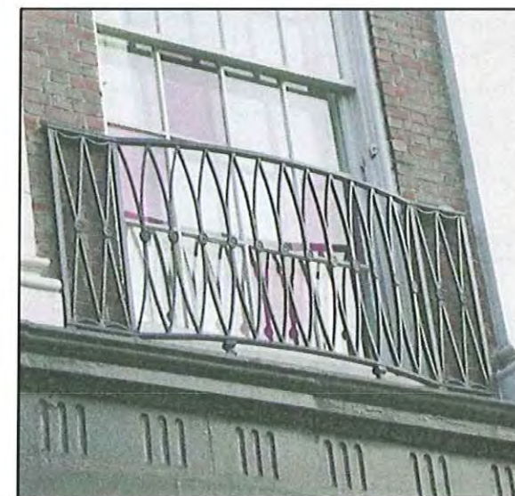
Painted Metal Railing
