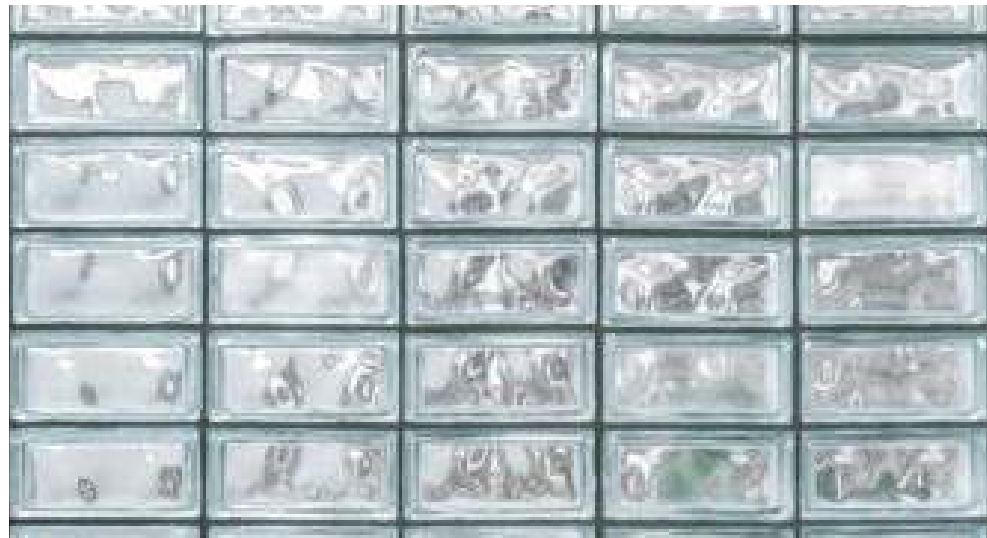
GLASS BLOCK - CLERESTORY WINDOWS AT BASE
