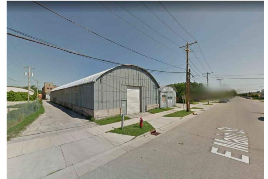
VIEW THREE LOOKING NORTH 827 E MAIN ST
