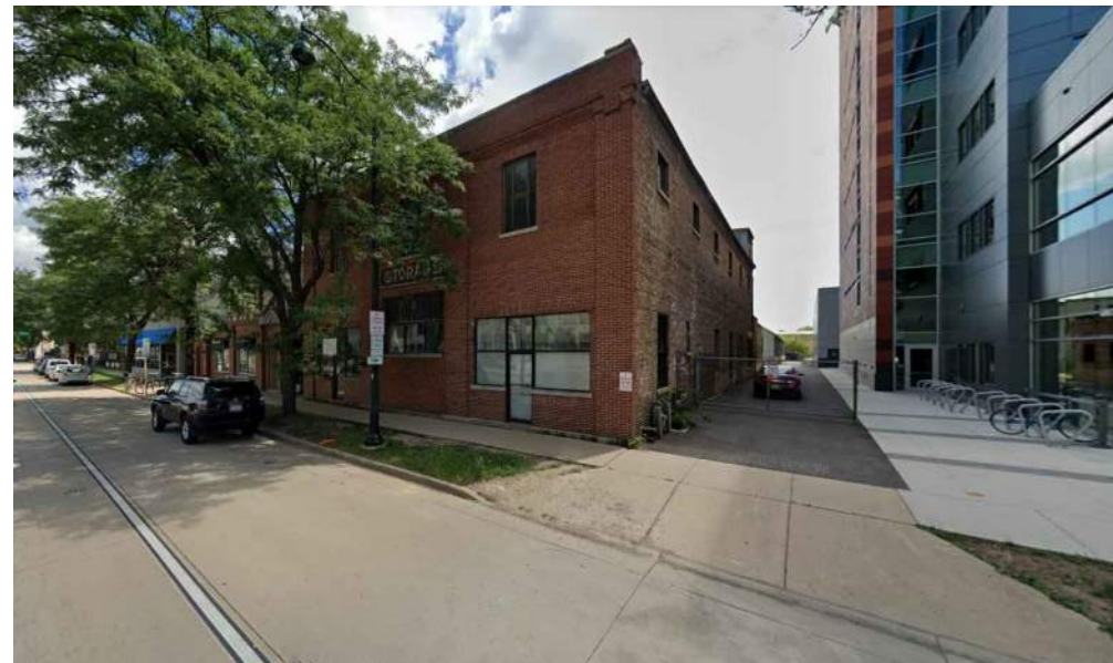
VIEW TWO LOOKING EAST 821 E. WASHINGTON AVE
