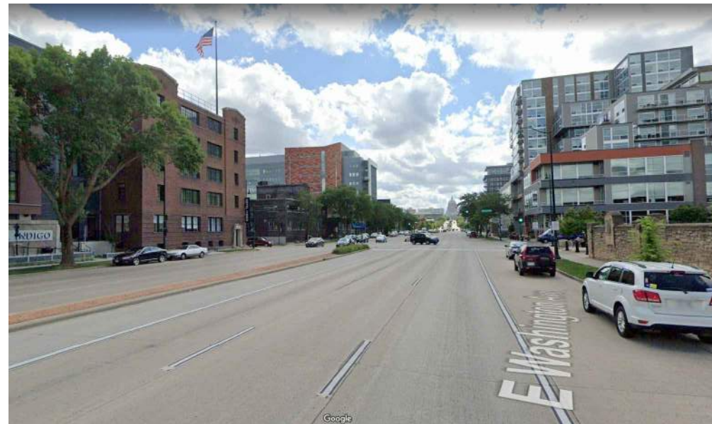
VIEW TWO LOOKING SOUTHWEST 901 E. WASHINGTON AVE
