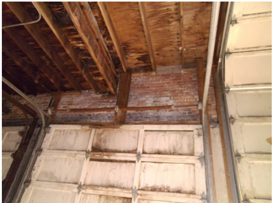
Images showing the interior and exterior surfaces of the east wall.
