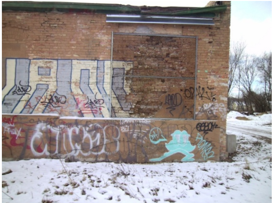
Image showing the west end of the north wall.
