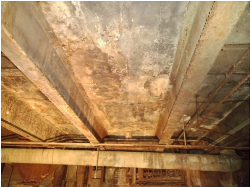
Image showing a portion the floor construction of second floor.
