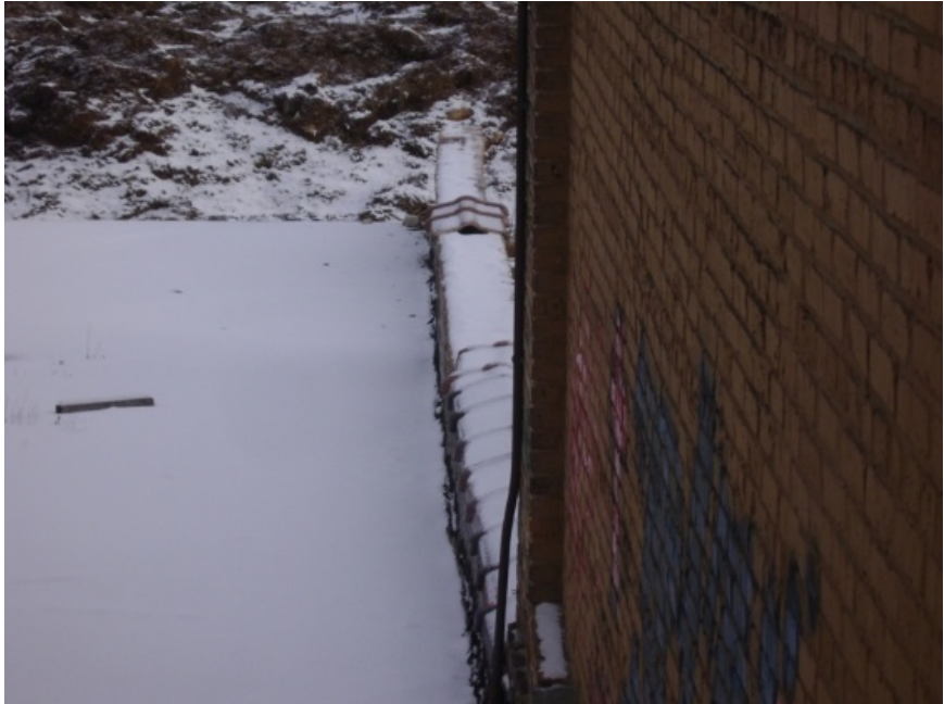
Image showing the sweeping curvature of the east wall.
