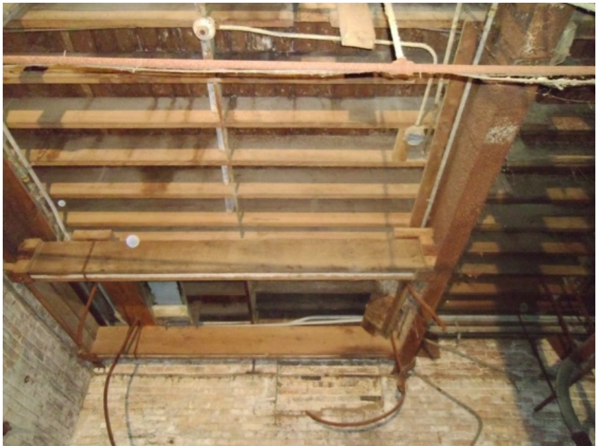
Image showing the floor construction of the second floor.
