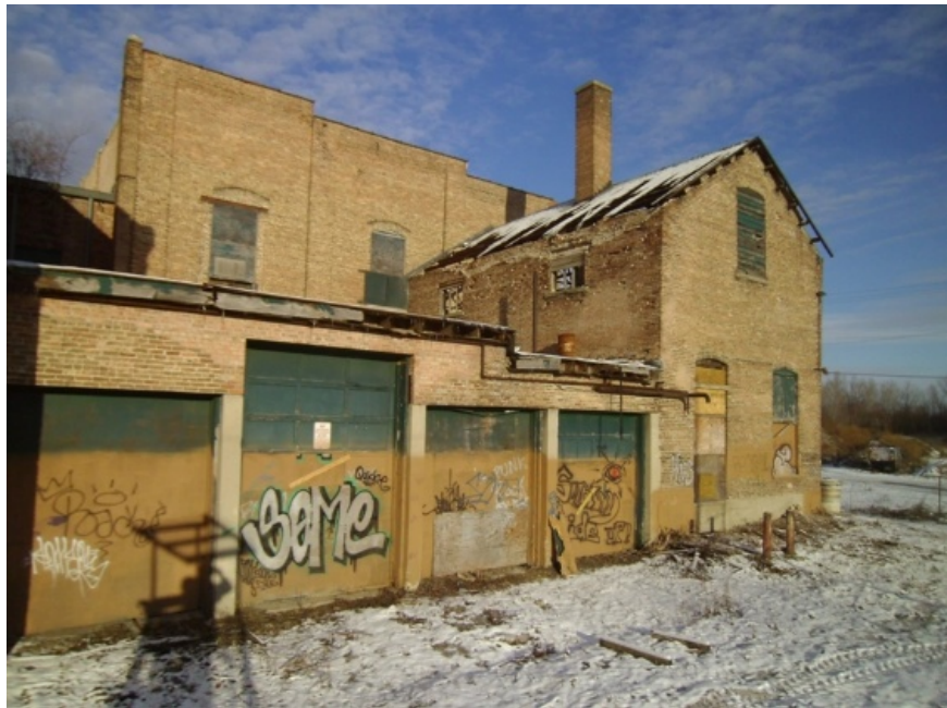
Image showing the east elevation of module C & D.
