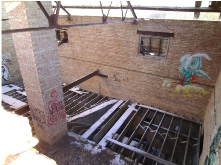
Image showing the brick chimney.
