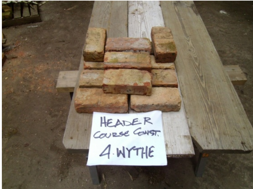
Image showing header course construction of four wythe wall.
