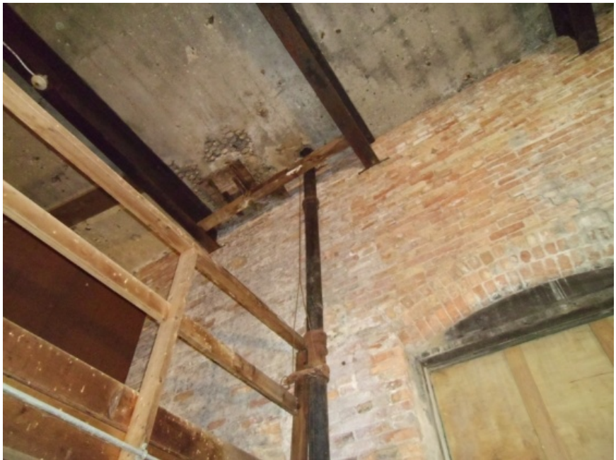
Image showing the bearing of steel beams into the masonry walls.
