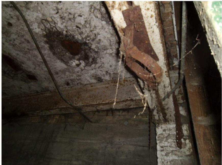
Images showing the pits/vaults below the first floor.
