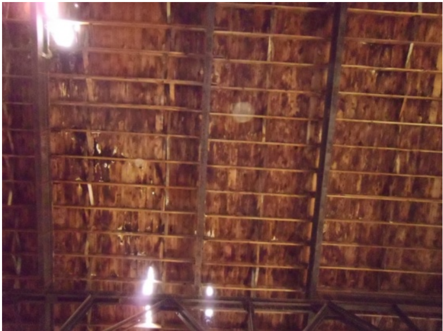
Image showing the construction of the existing wood and steel framing.
