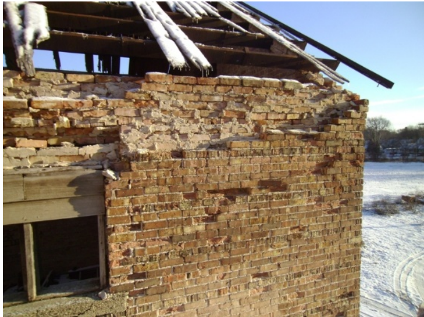
Image showing a section of the south wall.
