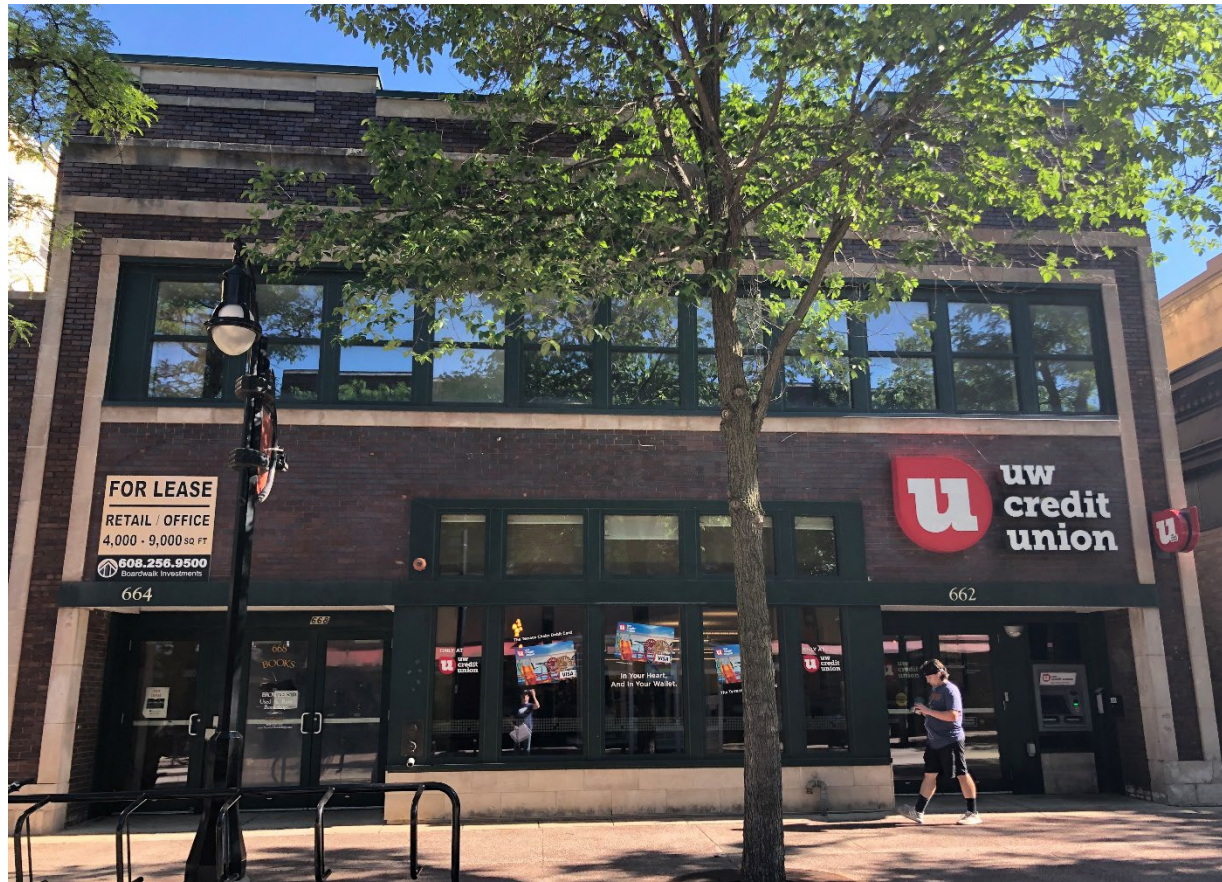
EXISTING PRESENTDAY PHOTOS (NORTH ELEVATION)
