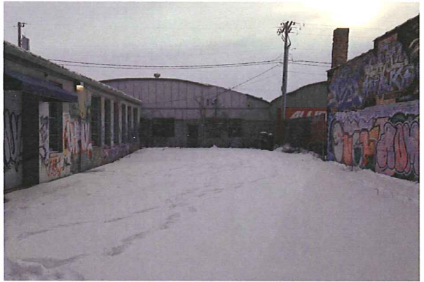
4 VIEW SOUTHEAST INSIDE COURTYARD
