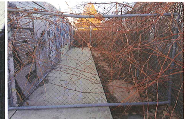
7 VIEW BEHIND EXISTING BUILDING
