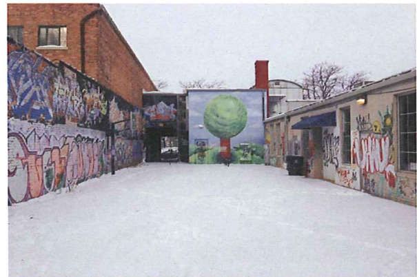
5 VIEW NORTHWEST INSIDE COURTYARD
