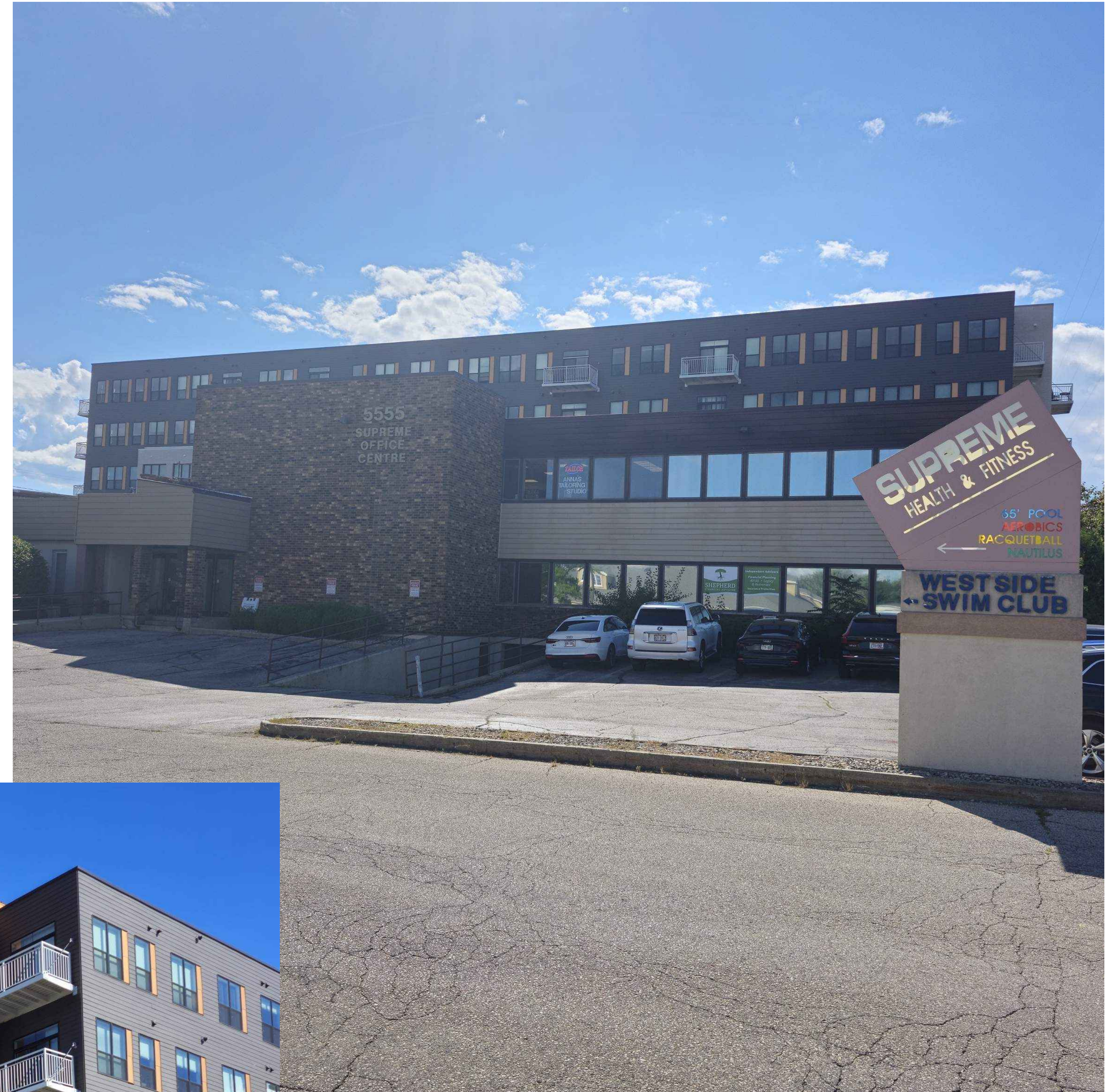
EXISTING BUILDING FROM ODANA ROAD LOOKING WEST
