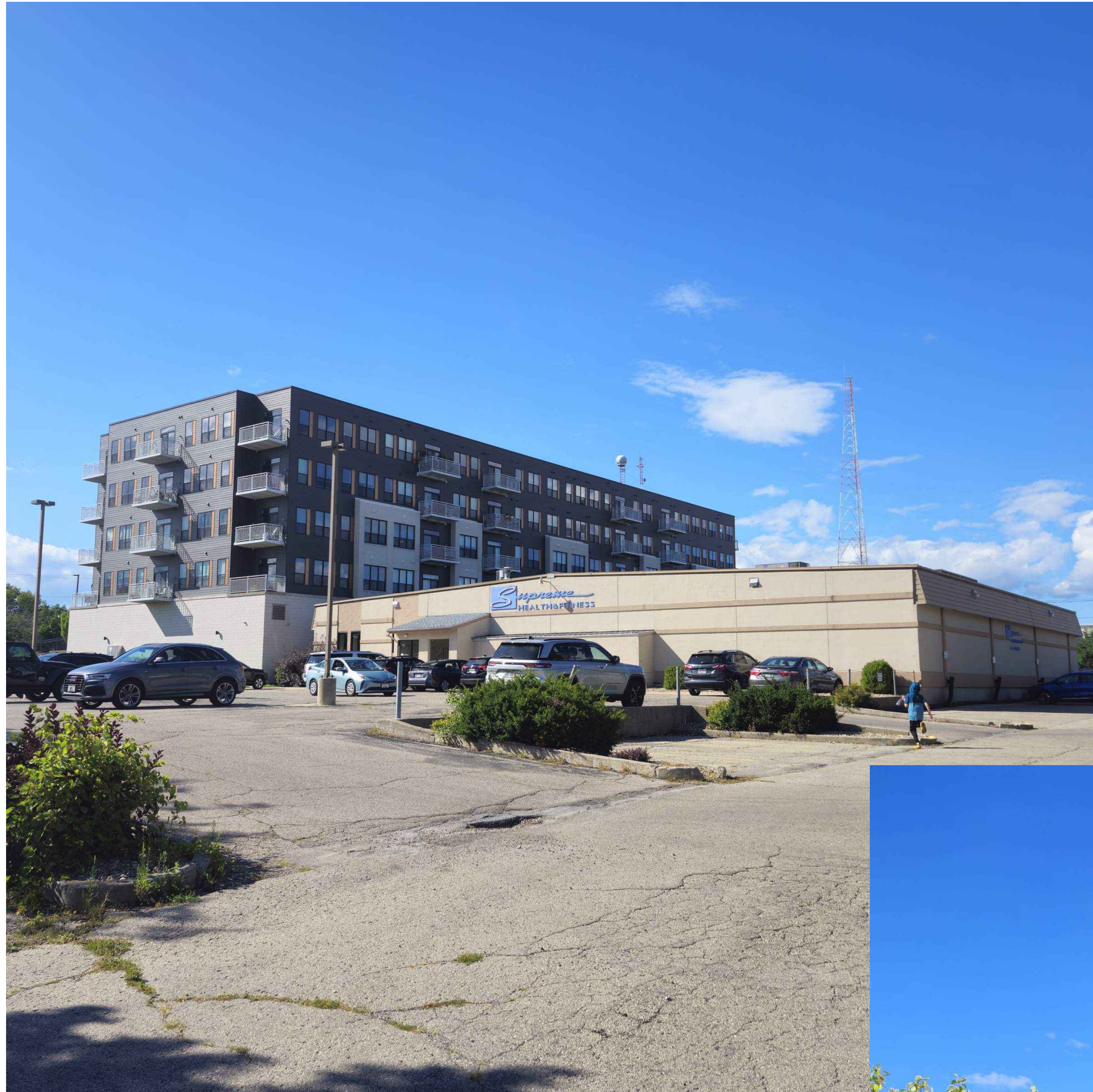
EXISTING BUILDING FROM CENTER OF PROPERTY
