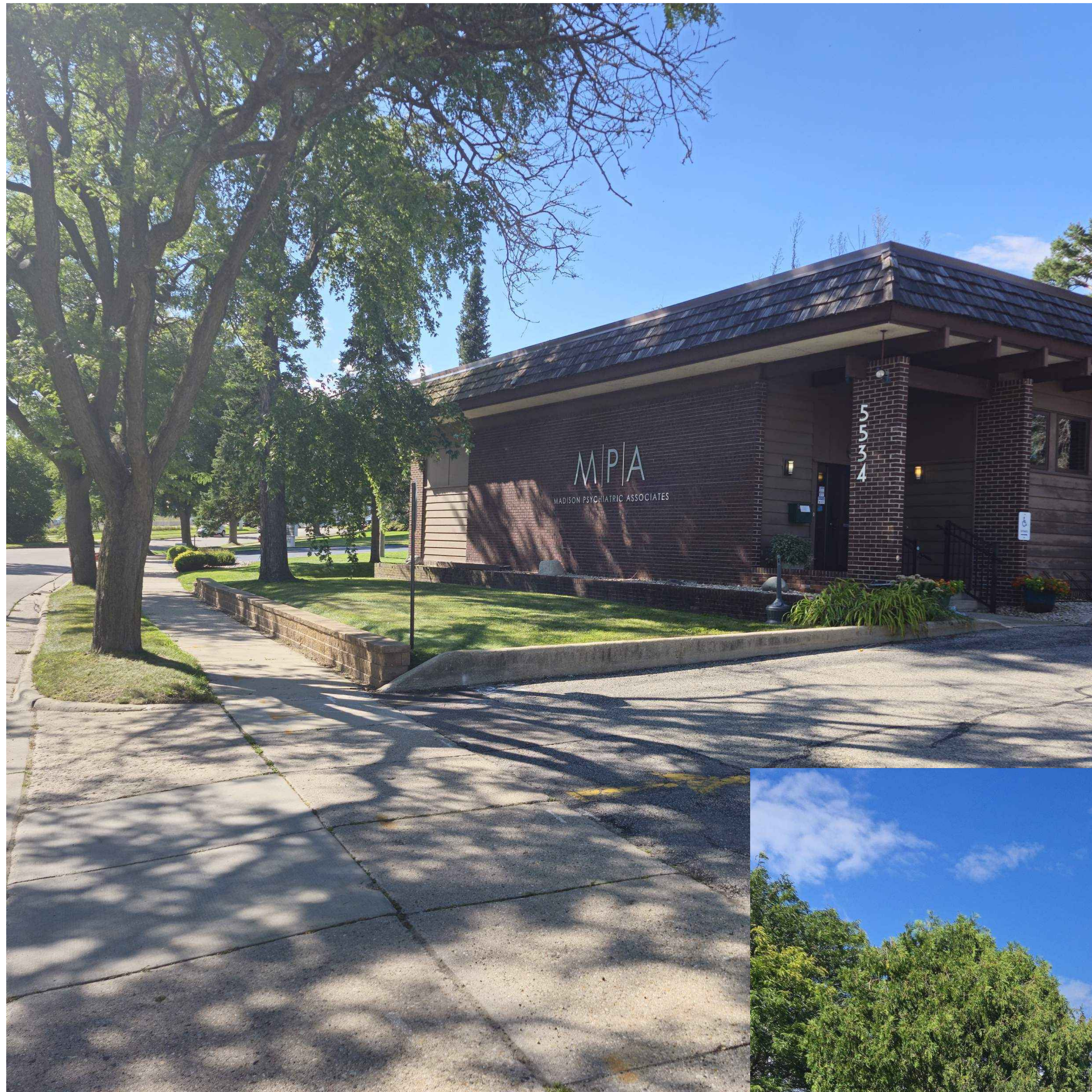
EXISTING BUILDING FROM MEDICAL CIRCLE LOOKING WEST
