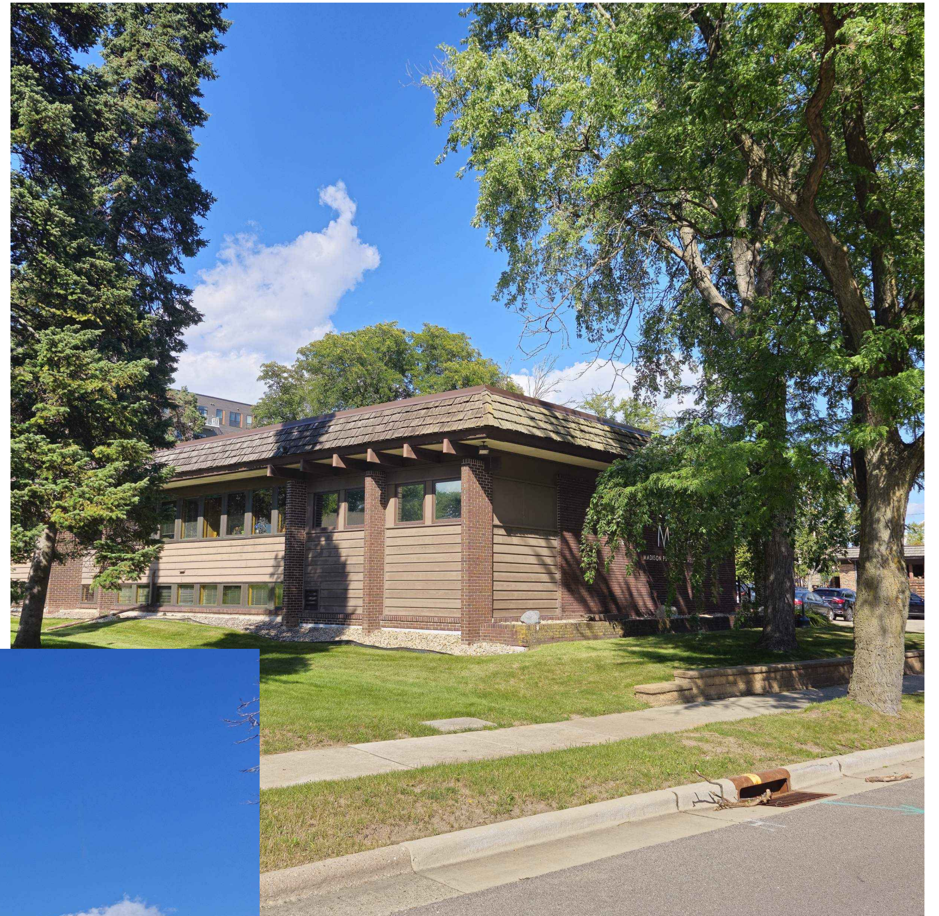
EXISTING BUILDING FROM MEDICAL CIRCLE LOOKING EAST
