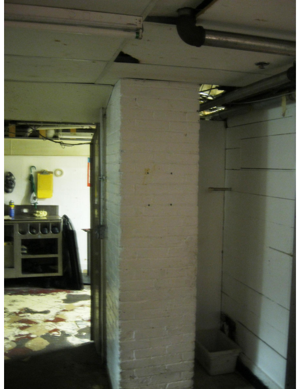
Photo 5 – Basement level brick pier
