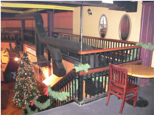
Figure 11. Second floor mezzanine with original balustrade.
