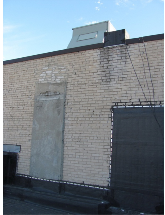
Figure 7. Left. Vertical cracking and localized damage in the brick masonry party wall, which is visible where it extends above the roofs of the adjacent buildings.
