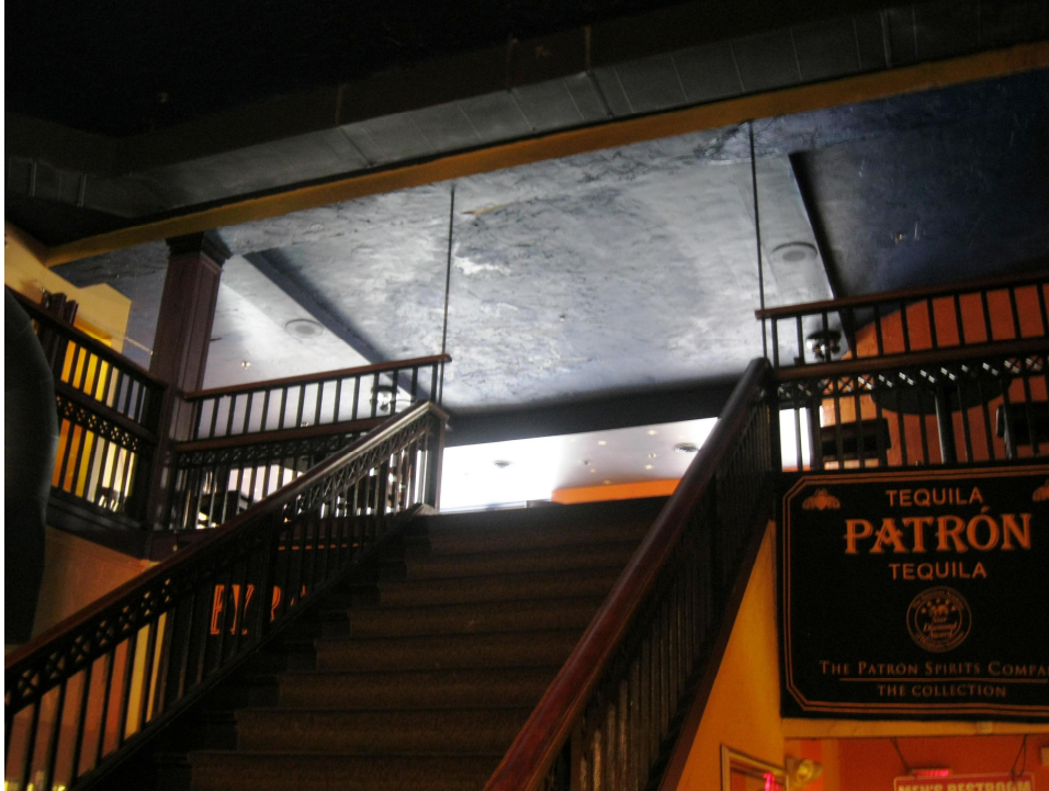
Photo 1 – 3 rd floor beams and column viewed from 1 st floor restaurant
