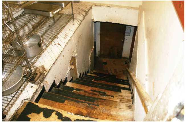
First Floor: View of access to basement
