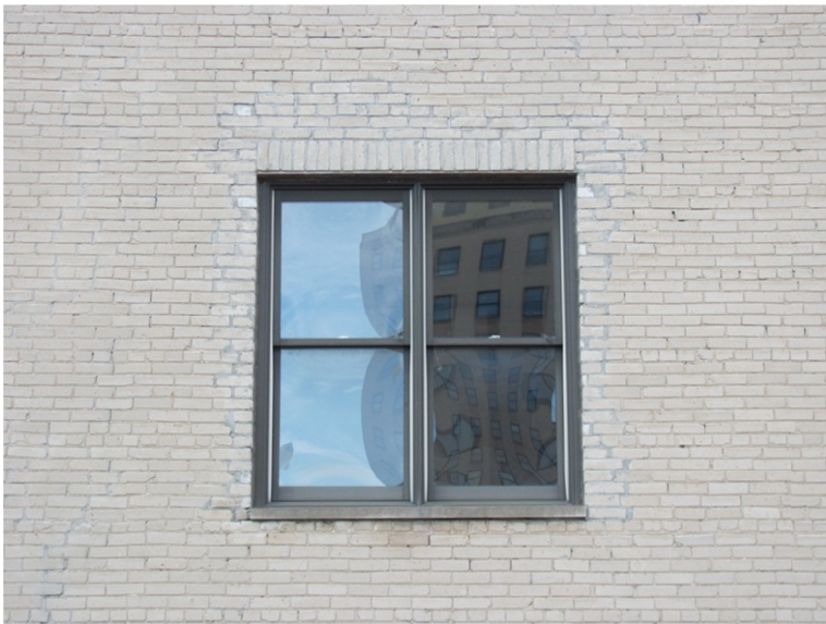
Figure 9. Typical aluminum-clad wood windows.
