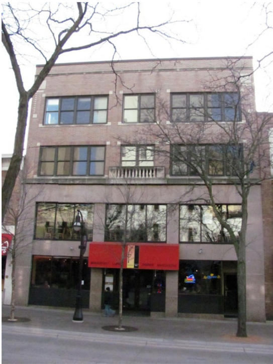
Figure 1. The State Street facade.
