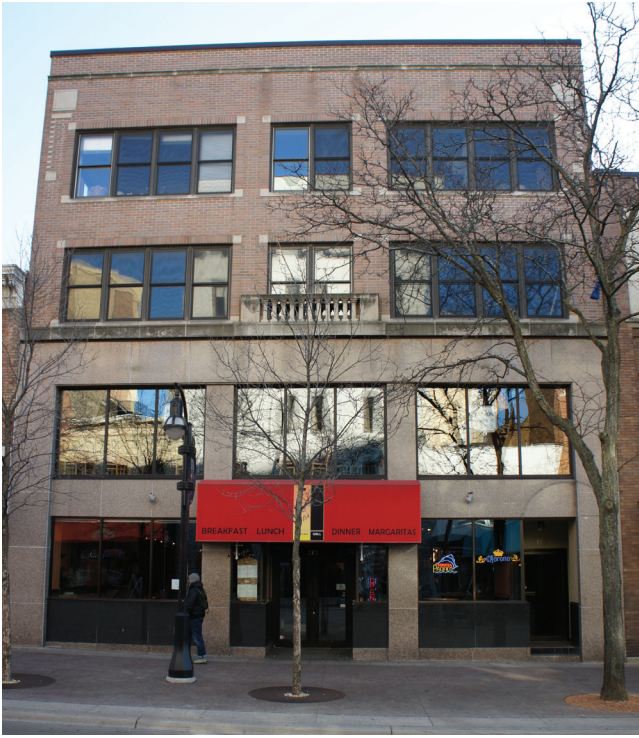
View of Front Facade
