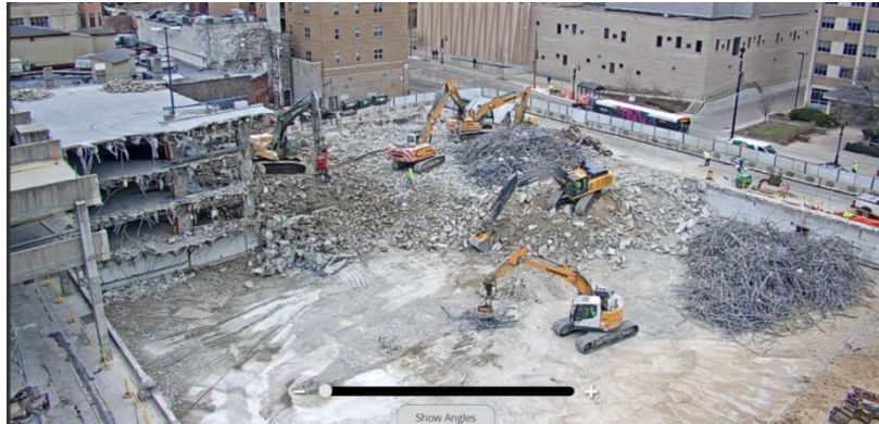
Figure 29 Demolition of State St Campus Garage Began in January 2024
