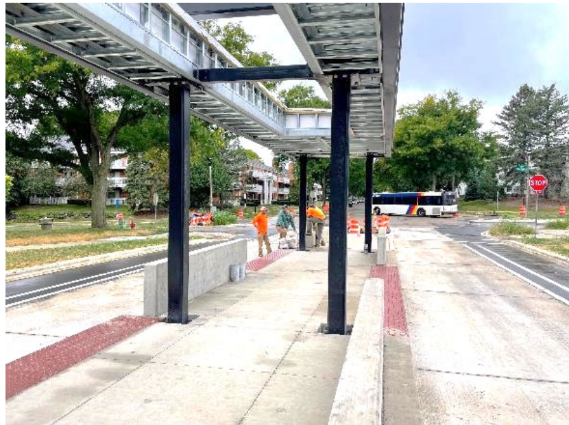
Figure 18 Eau Claire BRT Station Early Stages
