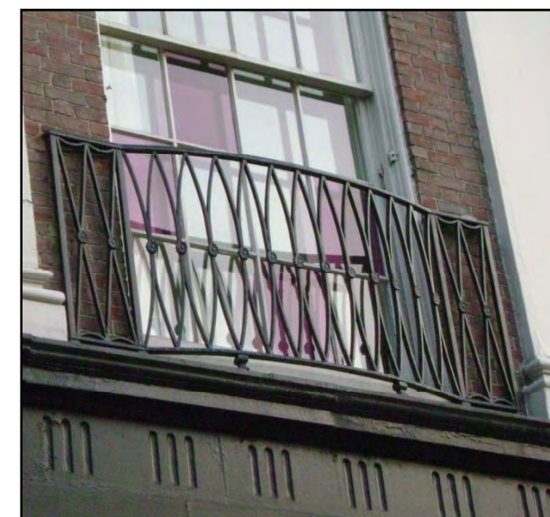
Painted Metal Railing
