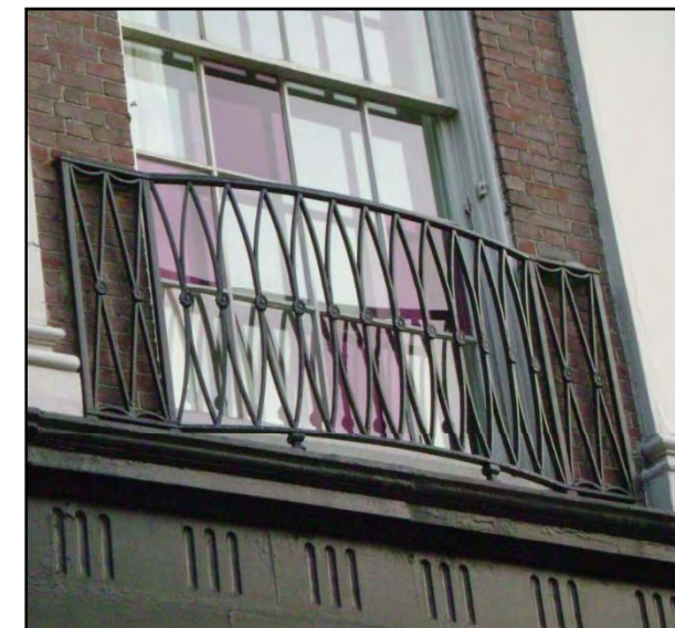
Painted Metal Railing
