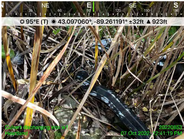
Photo #33 Photo of culvert discharging into W-1
