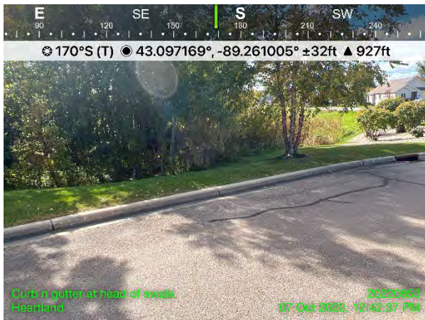
Photo #35 Photo of curb and gutter at head of swale (2 of 2)
