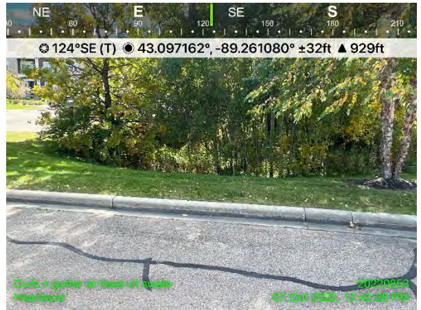
Photo #34 Photo of curb and gutter at head of swale (1 of 2)
