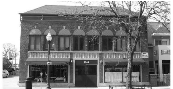
Figure K14: Typical Commercial Block Building Photo 2
