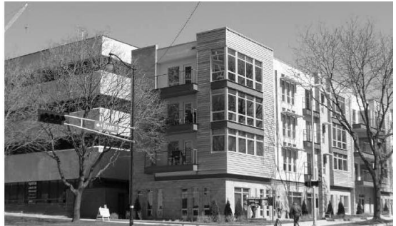
Figure K15: Typical Liner Building Photo
