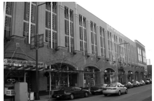
Figure K17: Typical Parking Building Photo
