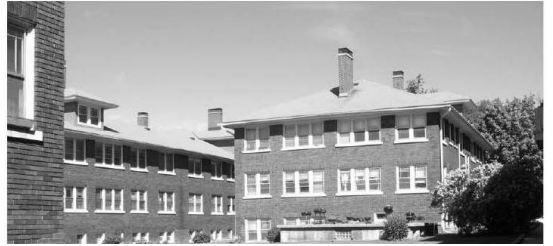
Figure K10: Typical Courtyard Multi-Family Building- Photo 1
