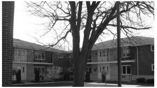
Figure K11: Typical Courtyard Multi-Family Building- Photo 2
