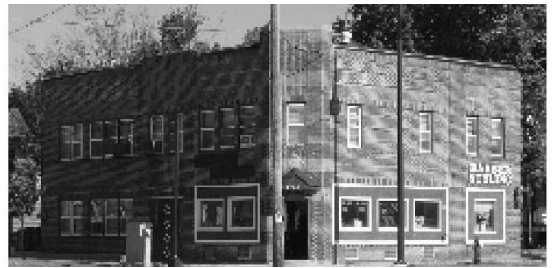
Figure K13: Typical Commercial Block Building Photo 1
