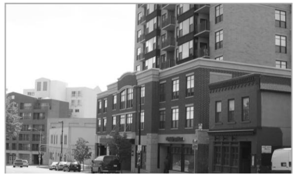
Figure K22: Typical Podium Building Photo
