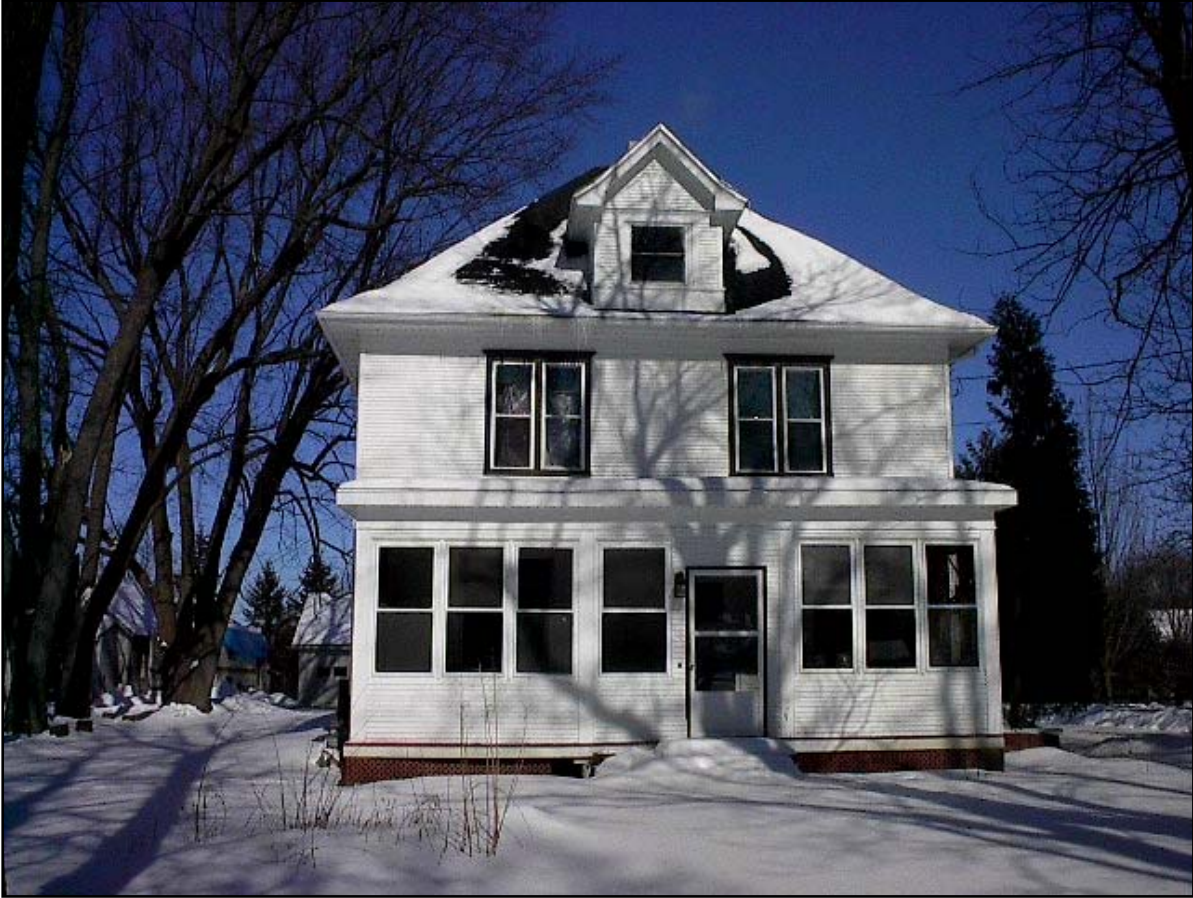
4. South Elevation – Faces Old Sauk Road
