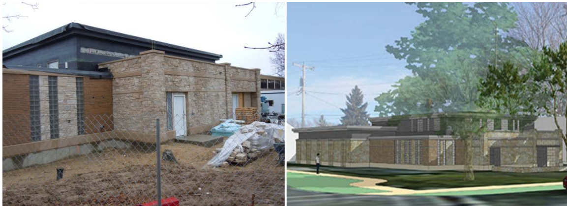
LEFT: WELL 7 UNDER CONSTRUCTION, DECEMBER 2014. RIGHT: ARCHITECTURAL RENDERING OF COMPLETED FACILITY.
