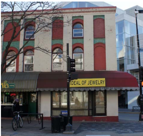
127-129 State Street, Francis Vallender Building State and Fairchild Street construction
