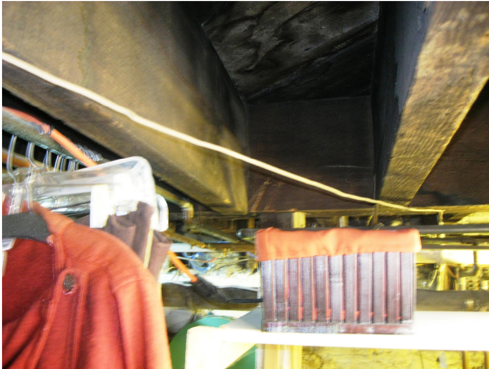
Photo 5 – 1 st floor joist framing
