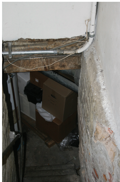
Basement Access Stair
