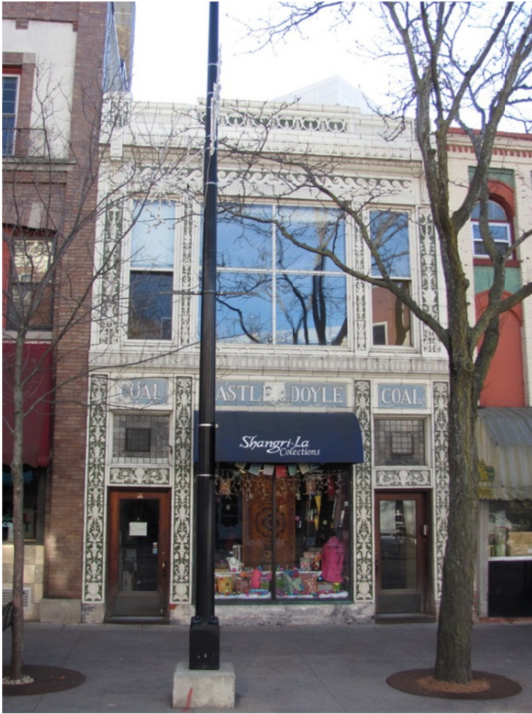
Figure 1. Overall view of the State Street facade.
