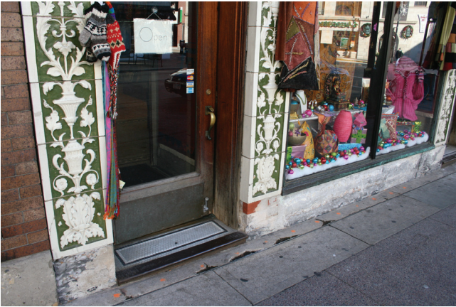
Exterior: View of entry stoop to first floor retail
