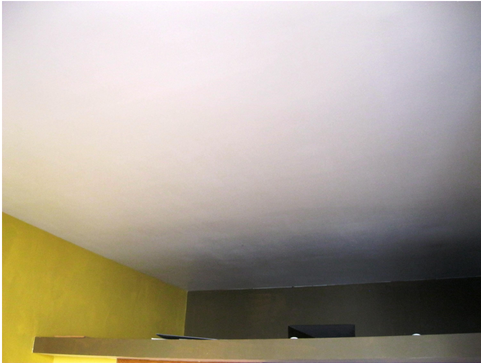
Photo 8 – 2 nd floor apartment ceiling
