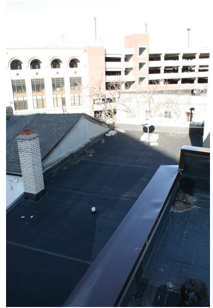
Exterior: View of roof
