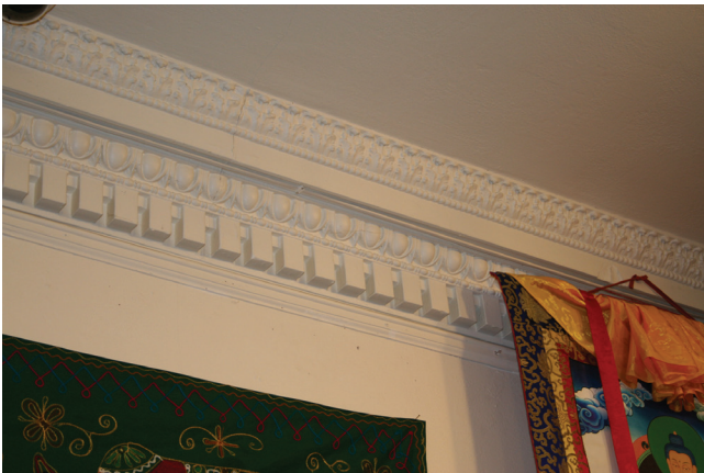
First Floor: Ceiling cornice
