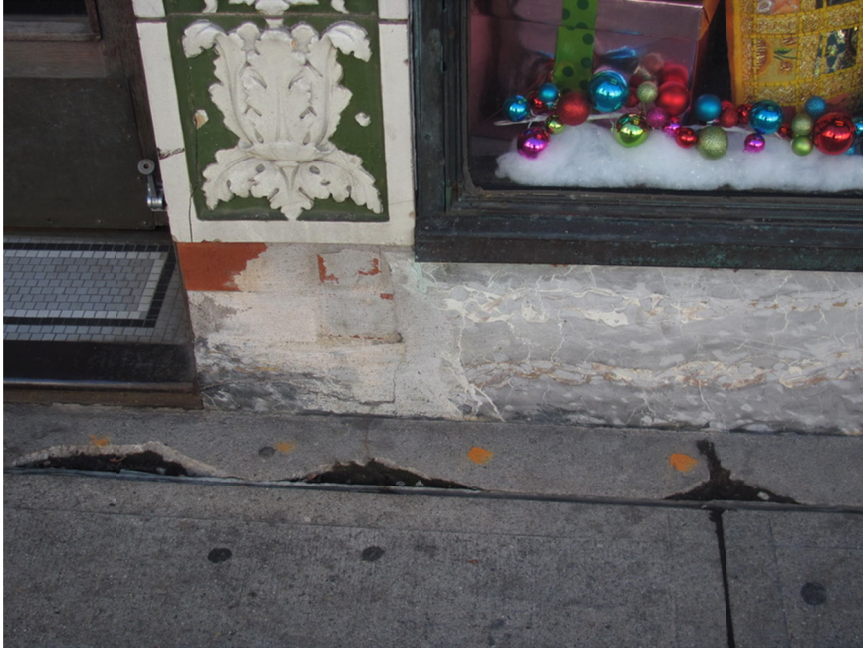
Figure 2. Marbleized cast stone and brick masonry at the base of the State Street facade.
