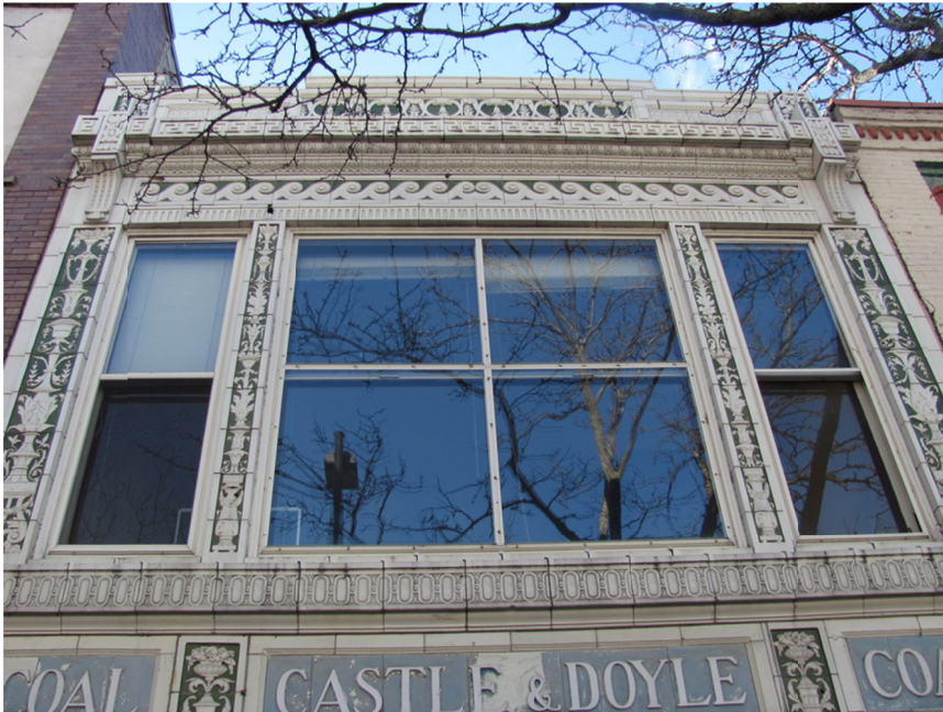
Figure 7. The central second floor window is a non-original assembly consisting of painted 2x wood framing supporting four panes of glass and a separate, similarly divided storm window.
