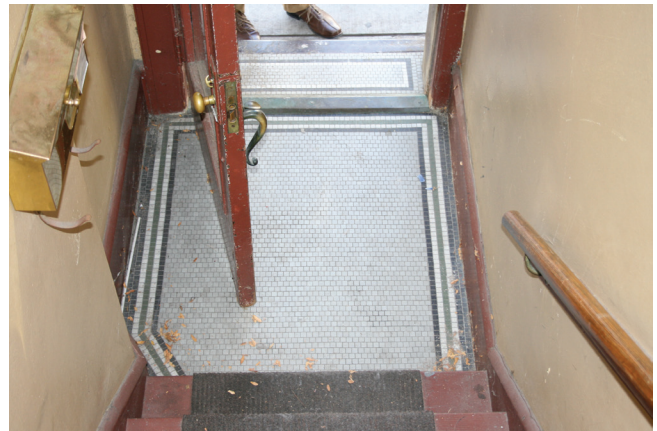
View of tile entry stoop from stairway to second floor
