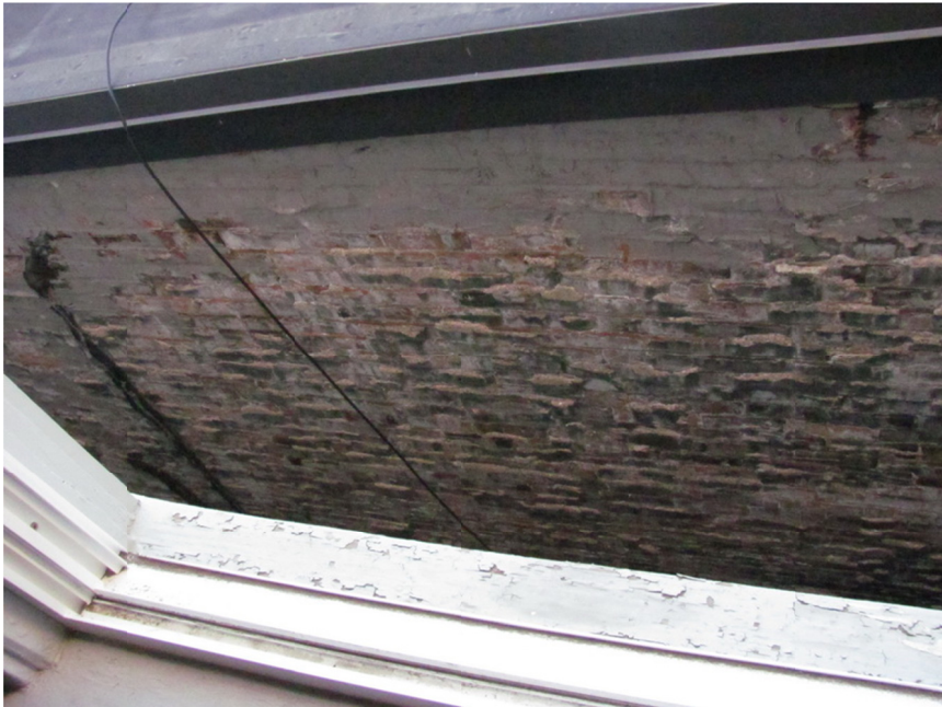
Figure 14. The masonry party wall as viewed from the adjacent building appeared to be in fair condition.
