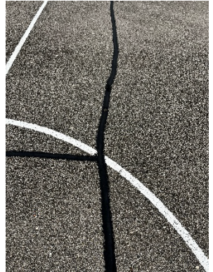
2025 Pavement Crack Sealing
