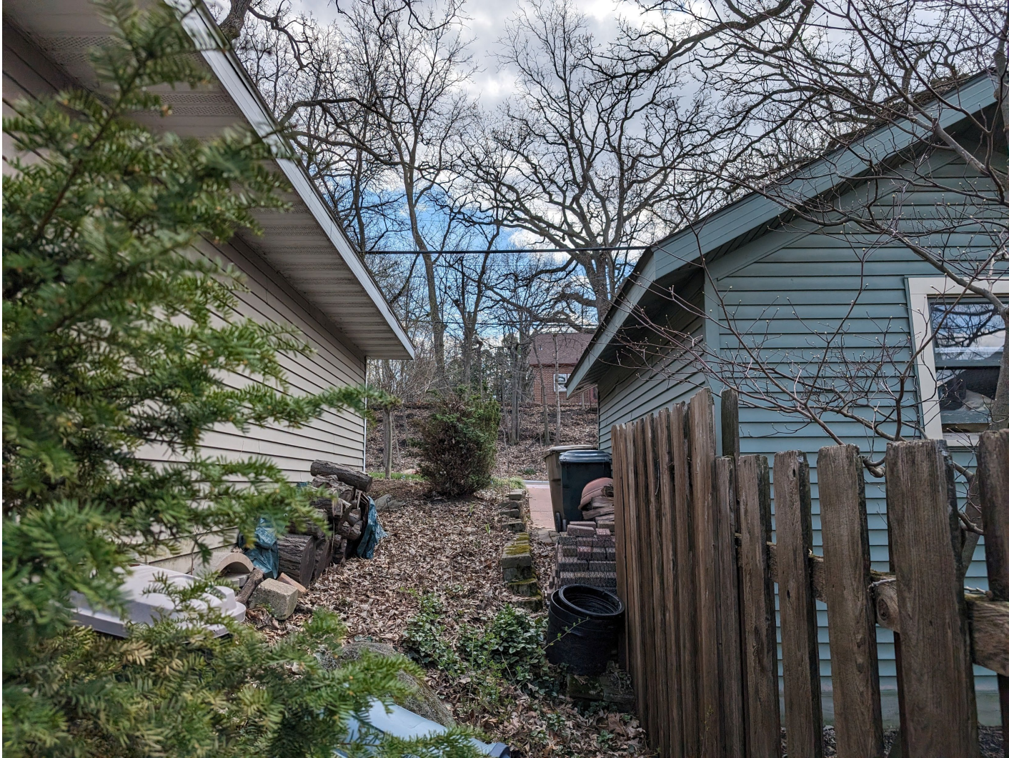
West Side Elevation, Looking Towards Lake Mendota Dr
