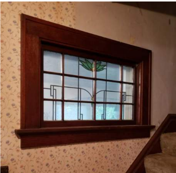
Historic Art Glass window - to be salvaged and reused. (this is a keeper!)
