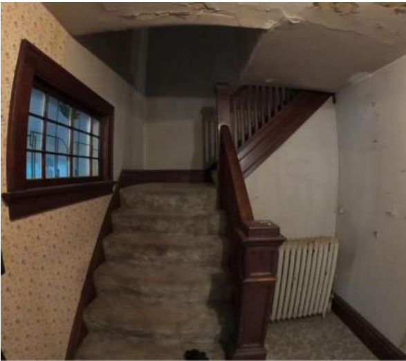
Existing Stair – limited 72” head clearance
