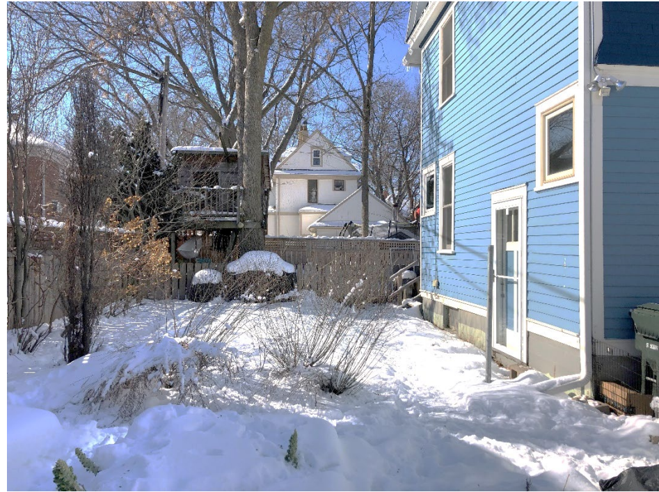
BACKYARD AREA, LOOKING WEST, GARAGE AND COVERED ROOF TO THE RIGHT
