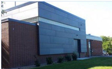
Municipal Well 15 PFAS Treatment Project Design of PFAS treatment facility at Well 15 to remove PFAS, PCE and TCE. Total project costs (estimate)*: $5.9M
