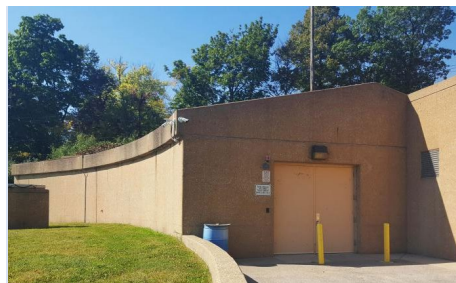
Municipal Well 19 Well Treatment Project Treatment facility at Well 19 to remove iron, manganese, and radium. Total project costs (estimate)*: $9.1 M
