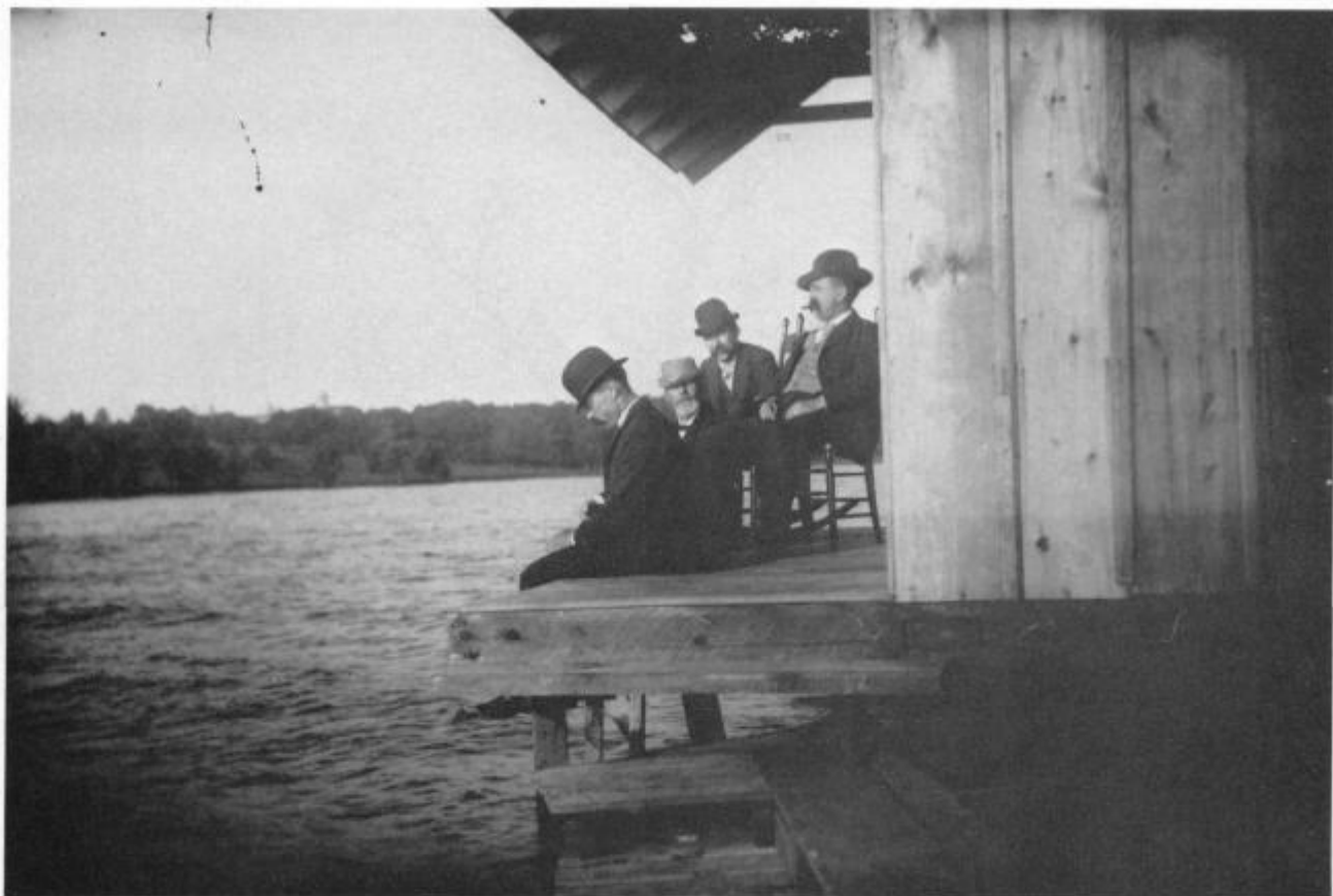
Newly built cottage on Rocky Roost, photographed September 18, 1892. Left to right: A. B. Morris, W. A. P. Morris, A. J. Dodge, and Melville C. Clarke (co-owner of the island with Robert M. Lamp), all prominent Madison businessmen. The unusual overhanging roof suggests Wright's influence, as do the porch and flagpole on the other cottage.
