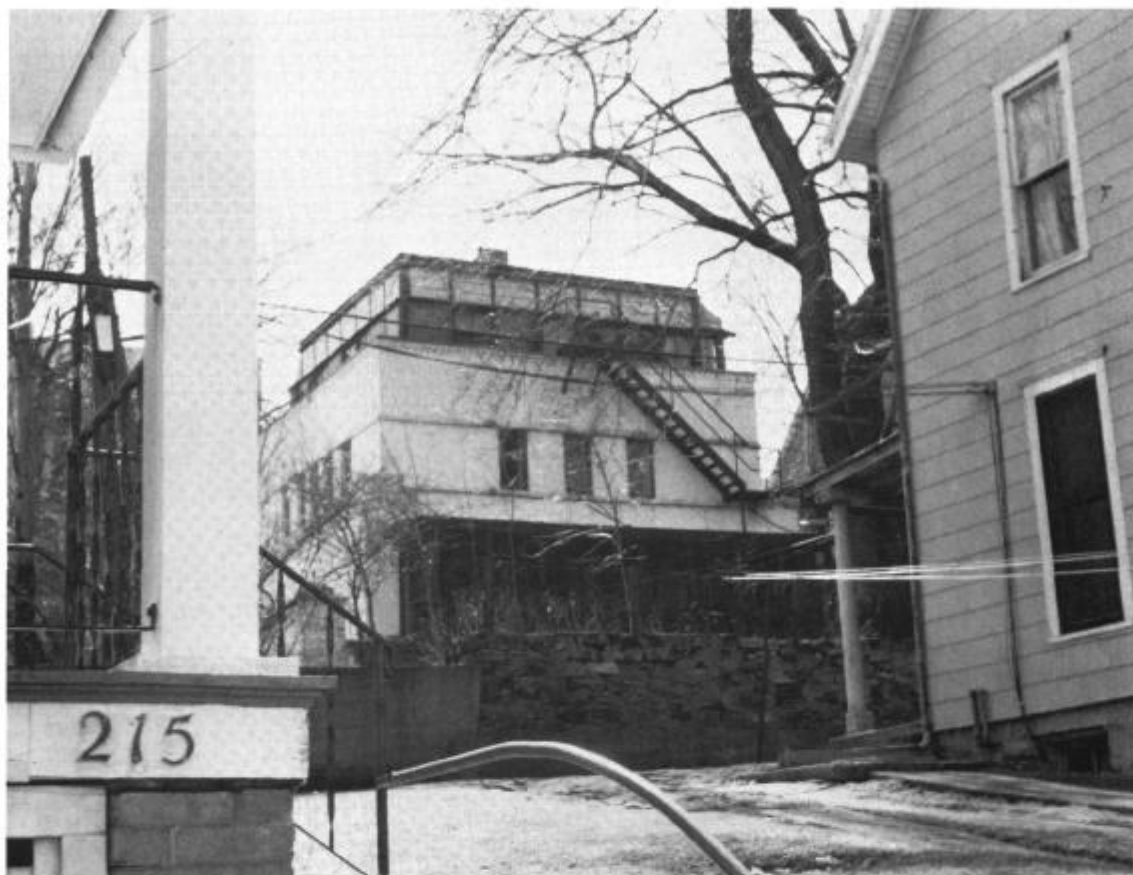
Late 1960's view from East Mifflin Street, the eastest angle from which to see the building. The fire escape was installed when the house was converted to apartments. WH(X3)35500
