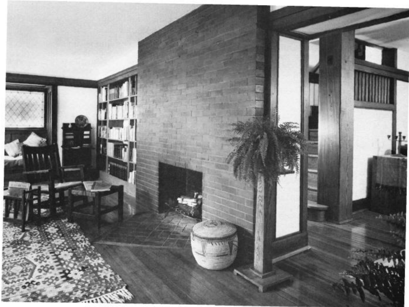
Lamp House living room with furnishings of the period. The bay window at the left was added during construction; the dining room is to the right. Woodwork is of red cypress; the upper band of woodwork originally ran across the fireplace as well. Bookcases are a reconstruction based upon the original drawings.
