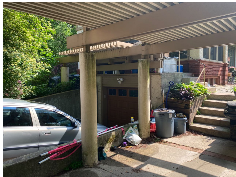
CARPORT LOCATION RESTRICTS ACCESS TO THE BACK DOOR OF THE HOUSE. WHEN A CAR IS PARKED HERE THE STAIRCASE ITAKING YOU DOWN FROM THE BACK DOOR POSITIONS YOU RIGHT INTO THE HOOD OF THE CAR.
