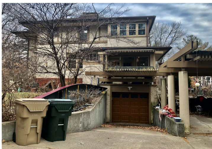
ORIGINAL SINGLE STALL GARAGE STALL AT BASEMENT LEVEL - TOO NARROW FOR MODERN CAR
