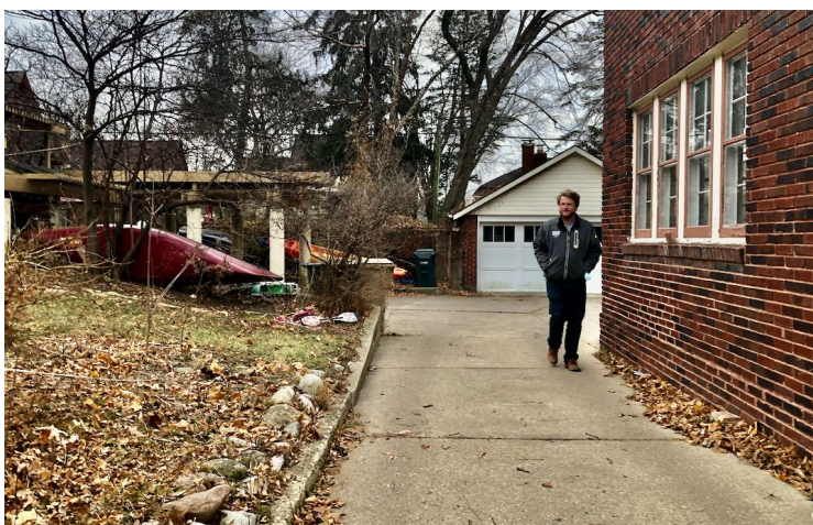
EXISTING 8'-6" WIDE DRIVEWAY TOUCHES THE NEIGHBOR'S HOUSE. WHEN THE CARPORT WAS INSTALLED THIS NECESSITATED USE OF THE NEIGHBOR'S DRIVEWAY IN ORDER TO ENTER AND LEAVE THE PARKING SPACE UNDER THE CARPORT. DESPITE NO NEIGHBOR OPPOSITION AT THE TIME THE CARPORT WAS APPROVED THIS OBJECTIVELY LIMITS THE NEIGHBOR'S FREE USE OF THEIR DRIVEWAY.
