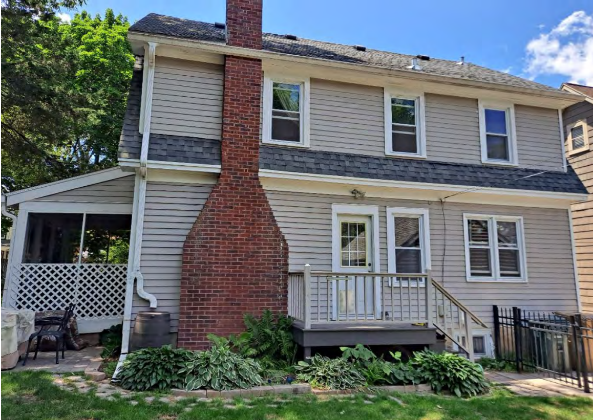
House - Existing Rear Elevation
