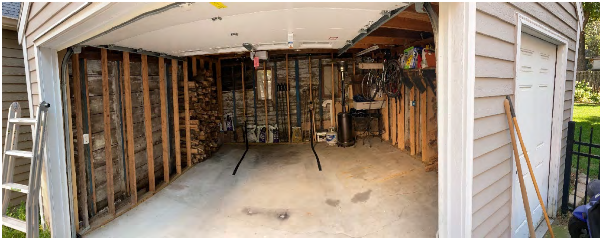
Garage Interior showing secondary structural support framing that restricts usable area.
