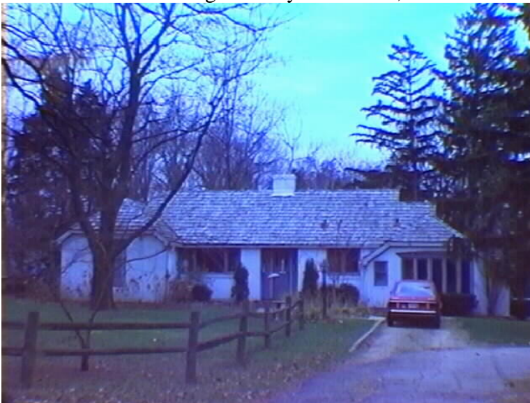
1202 Gilbert Road: single-family residential, built 1941
