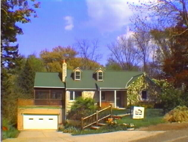
1119 Merrill Springs Road: single-family residential: built 1948
