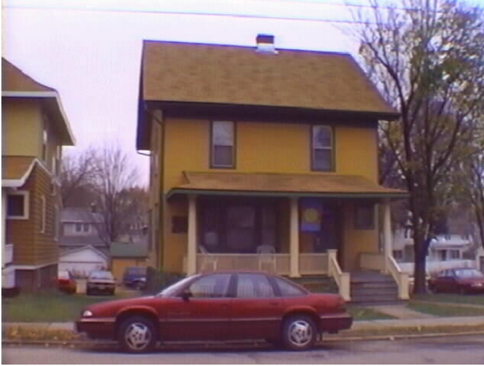
2021 Monroe Street: single-family residential: (badly damaged in fire)
